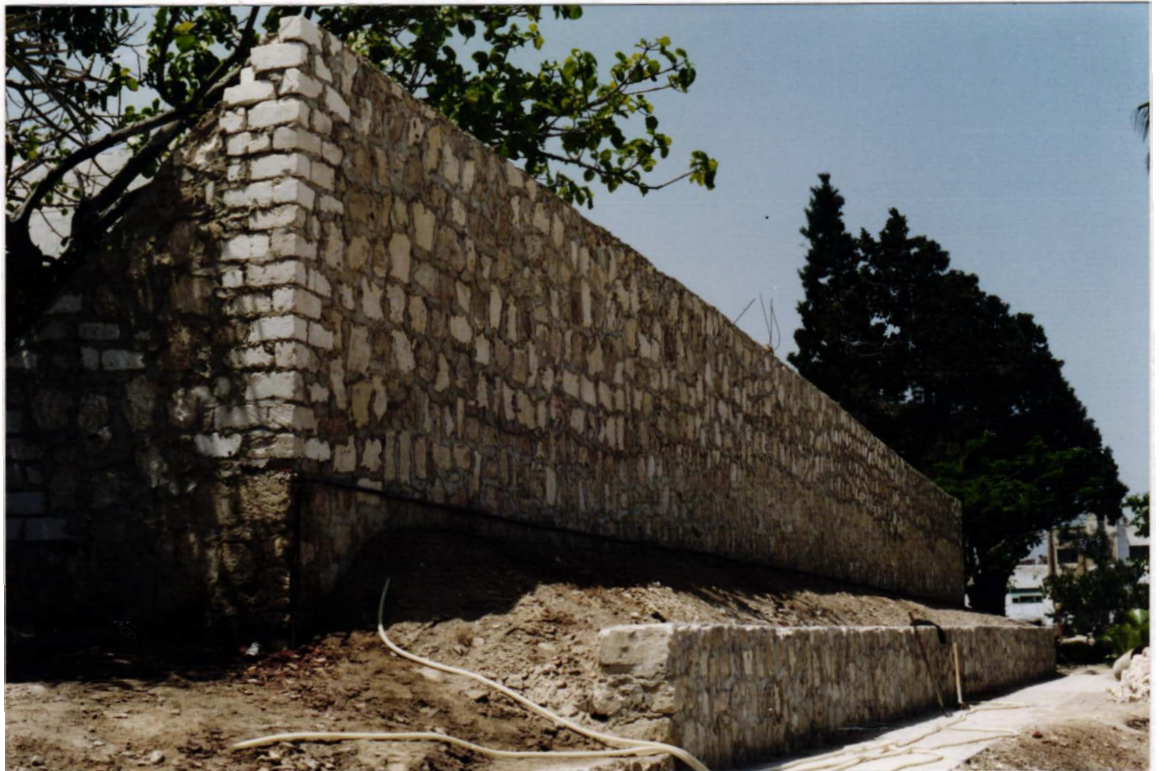
Phot. 11. Screening wall along the Fire Brigade area.
