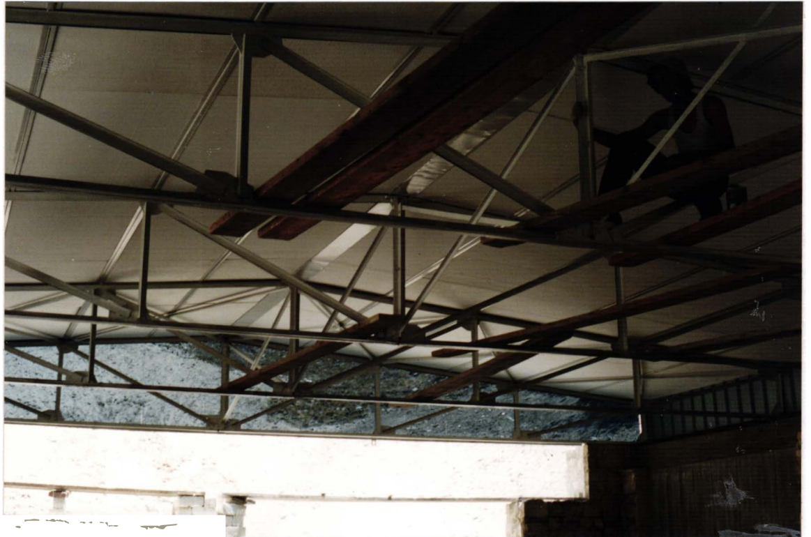
Phot. 9. Roof thermal insulation.
