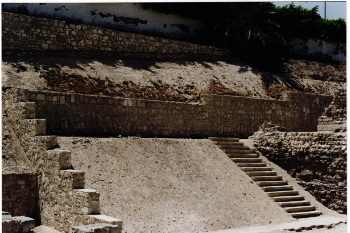
Phot. 10. Water supply pipe along the southern escarpment.
