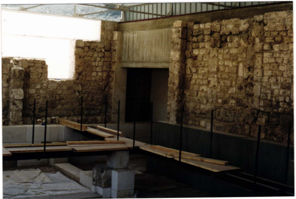
Phot. 1, 2. Foot-bridge construction.
