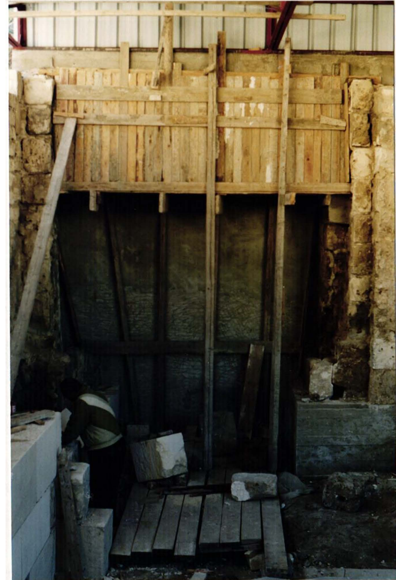
Phot. 7. Front wall above the ceiling; boarding.
