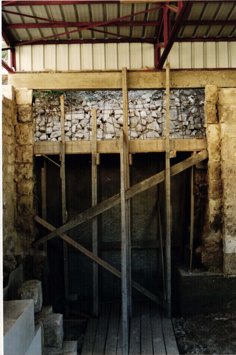
Phot. 6. Ceiling of the niche; boarding.
