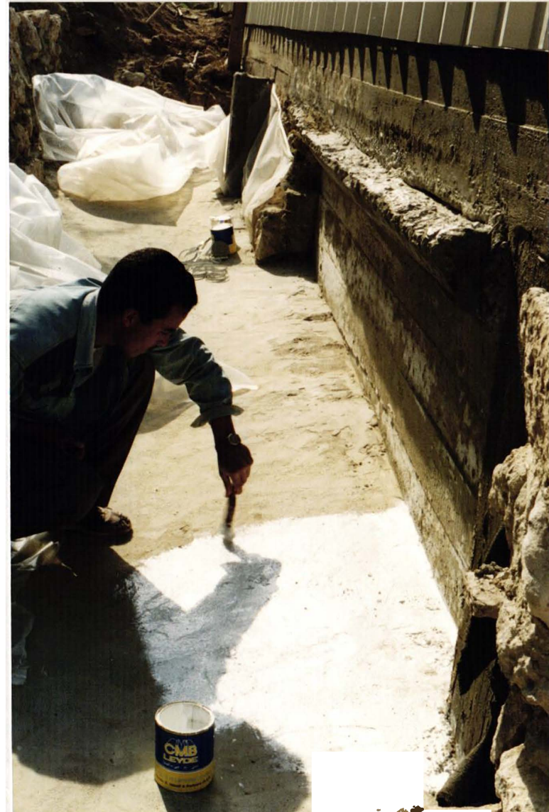
Phot. 13. Draining structure during insulation work.
