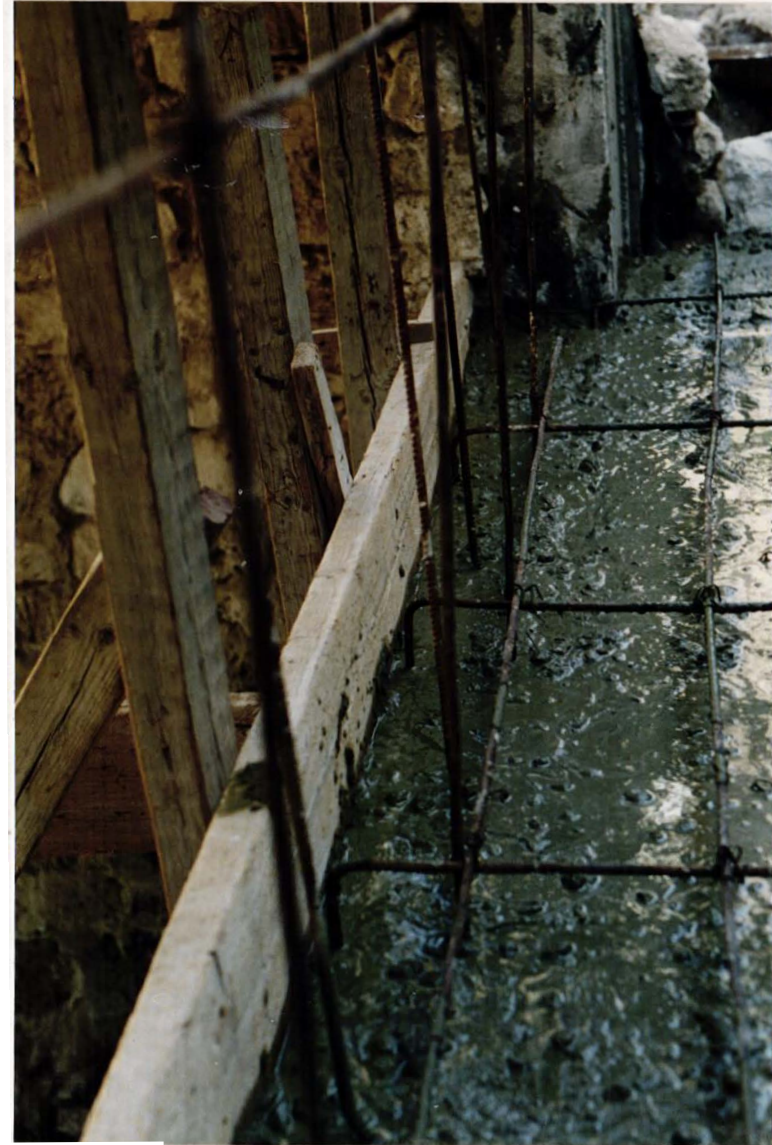
Phot. 9. Ceiling of the niche; placing concrete.
