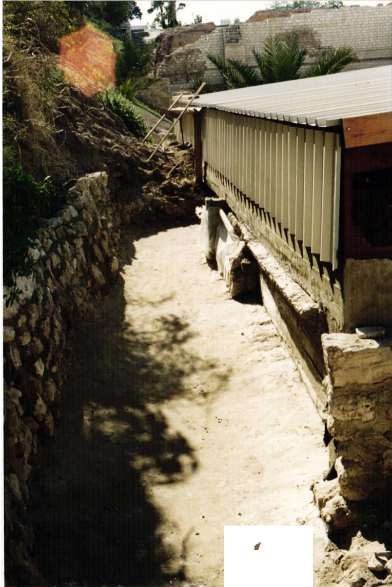
Phot. 12. Draining structure built above the ceiling.
