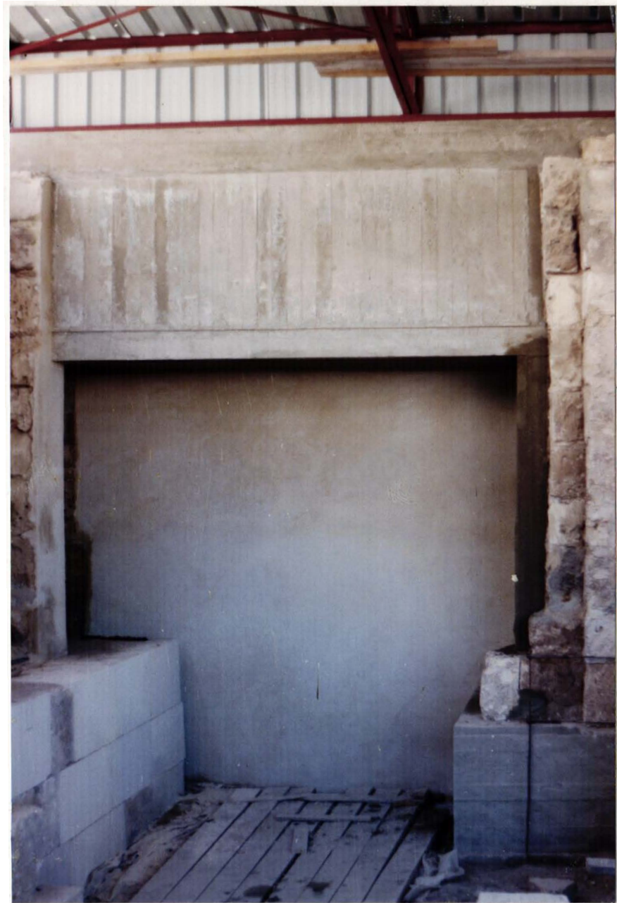
Phot. 11. The niche after completion of construction work.
