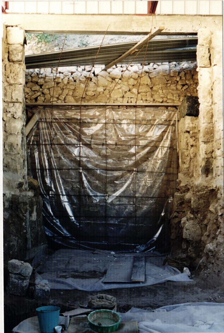
Phot. 4. Southern revetment wall; insulation and reinforcement structure.
