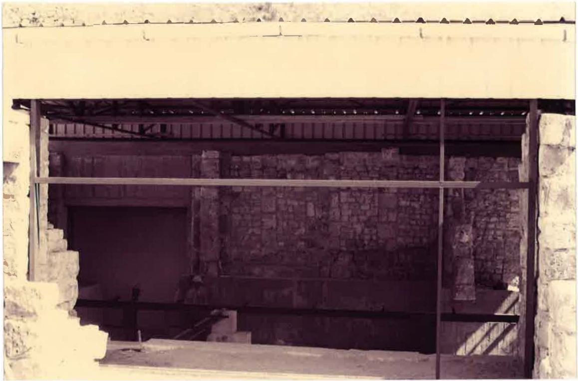
Phot. 18. Panel glass frames. Northern side of the shelter.
