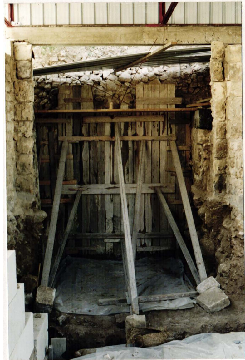
Phot. 5. Southern revetment wall; boarding.
