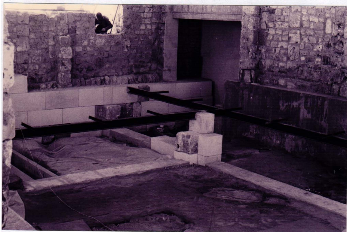
Phot. 16. Foot-bridge. General view.
