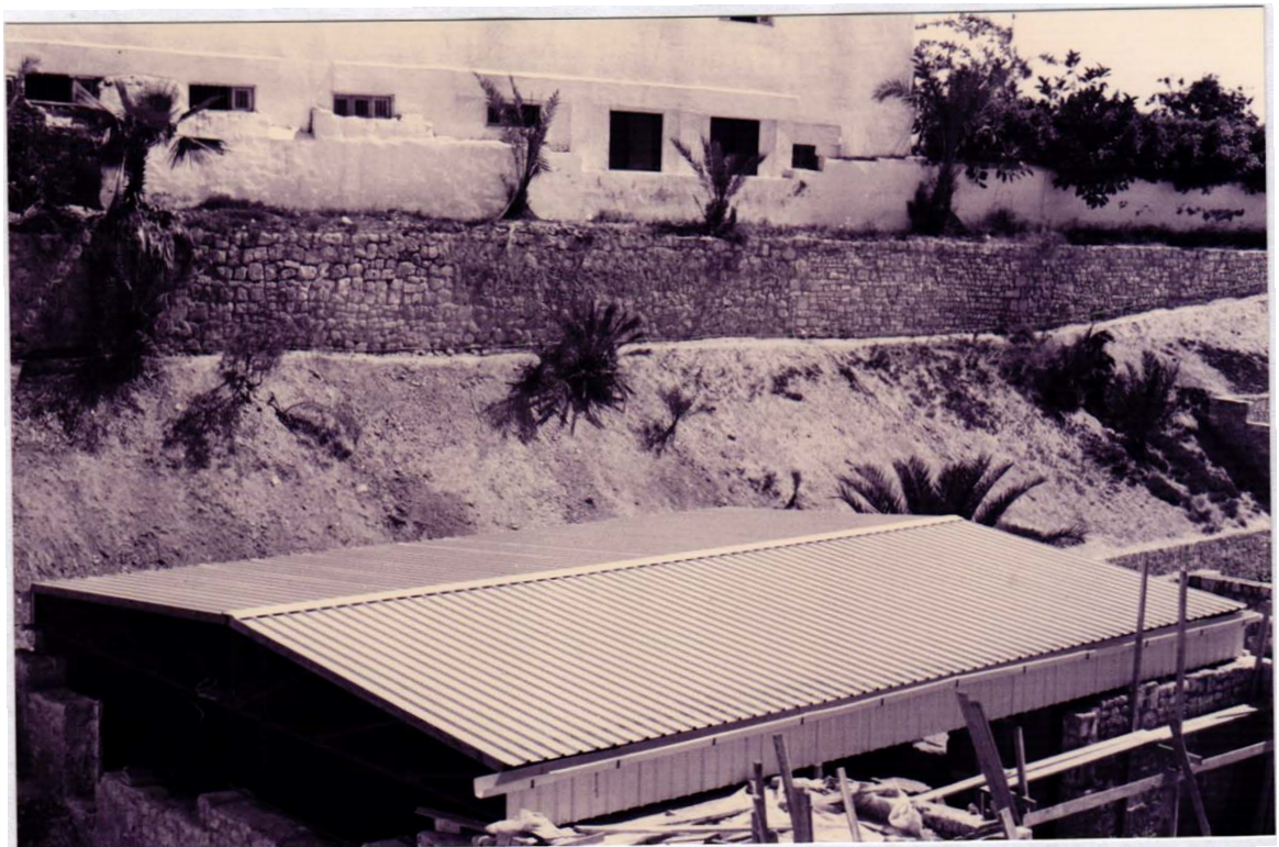
Phot. 15. Gutters along the northern edge of the roof.
