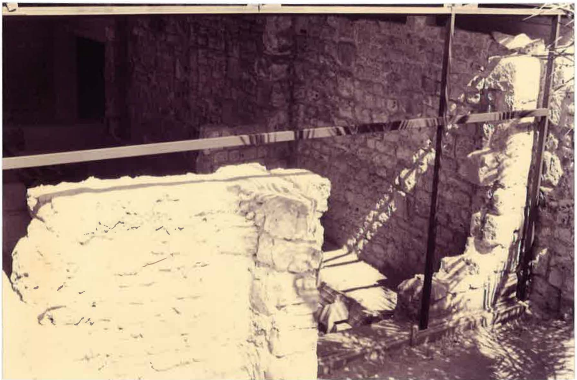
Phot. 19. Panel glass frames. Western side of the shelter.
