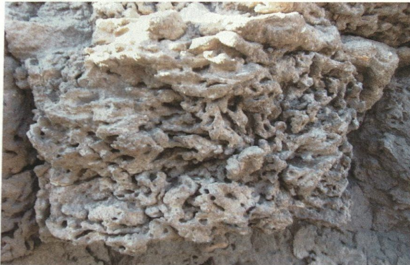
Figure 22: Detail of a typical mud brick that has these same surface decay patterns through its matrix.
