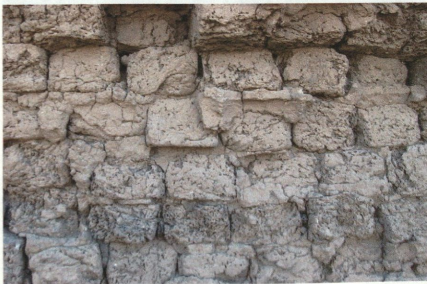
Figure 8: A detail of the individual mud bricks.
