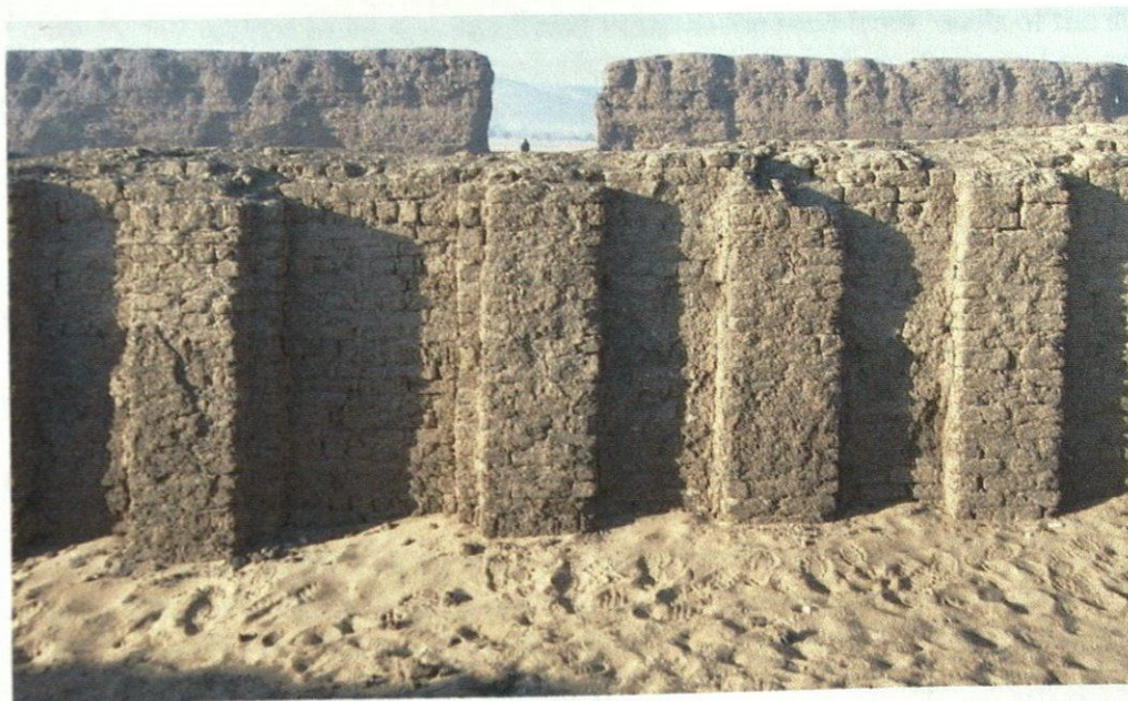
Figure 16: Pilasters on the east side of the east wall.
