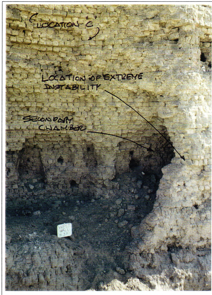
Photograph No. 78 Location "C" Monastic Cell
