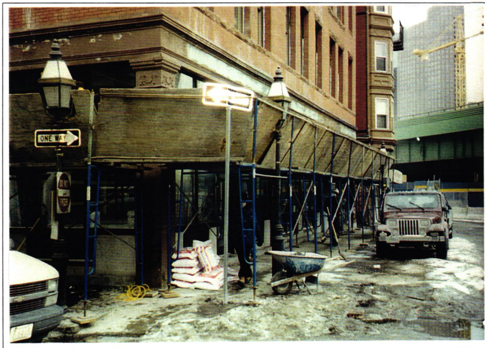
Photograph No. 44 Scaffold Protection at Modern Site
