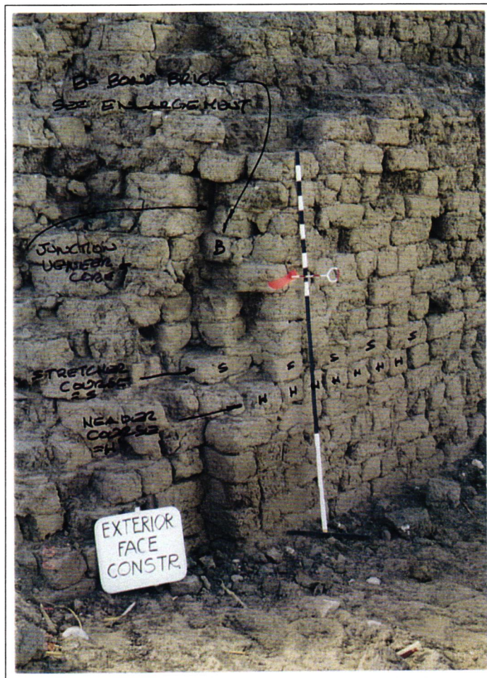
Photograph No. 5 Veneer and Core Wall Coursing
