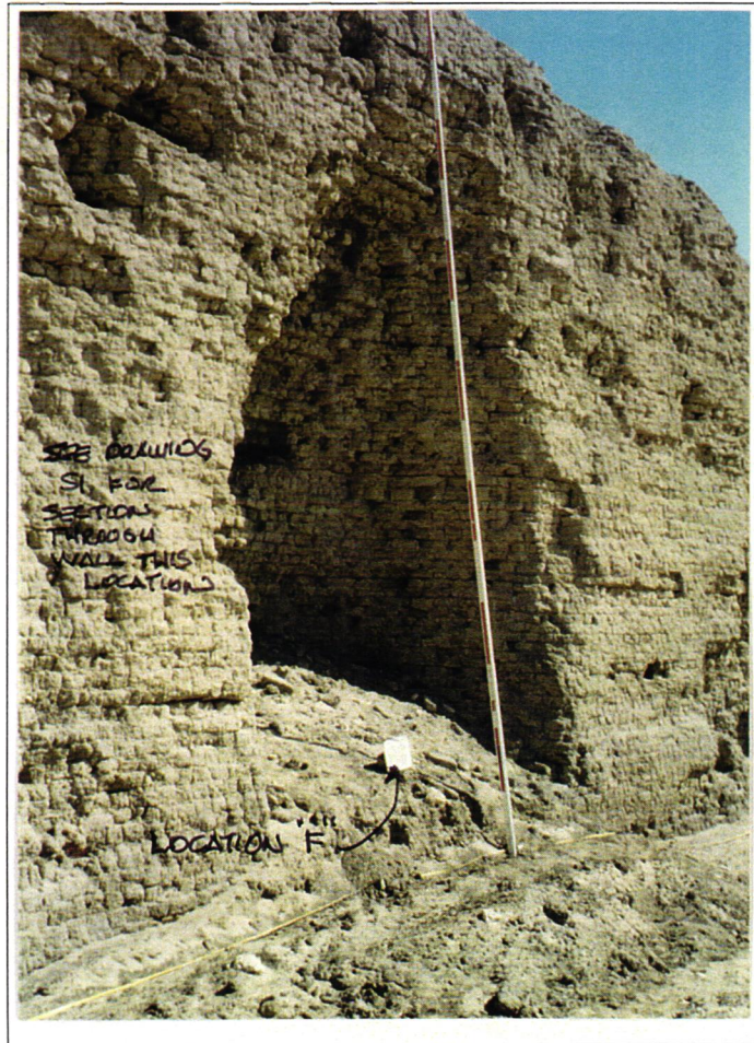
Photograph No. 98 Location "F" West Main Enclosure Wall
