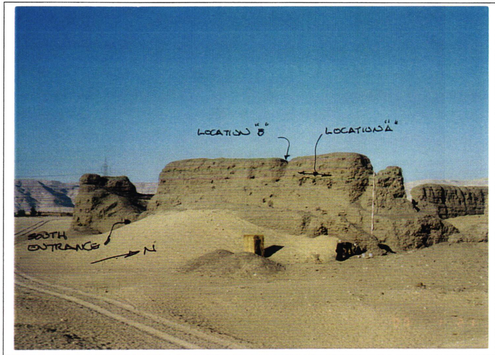
Photograph No. 113 South Main Enclosure Wall
