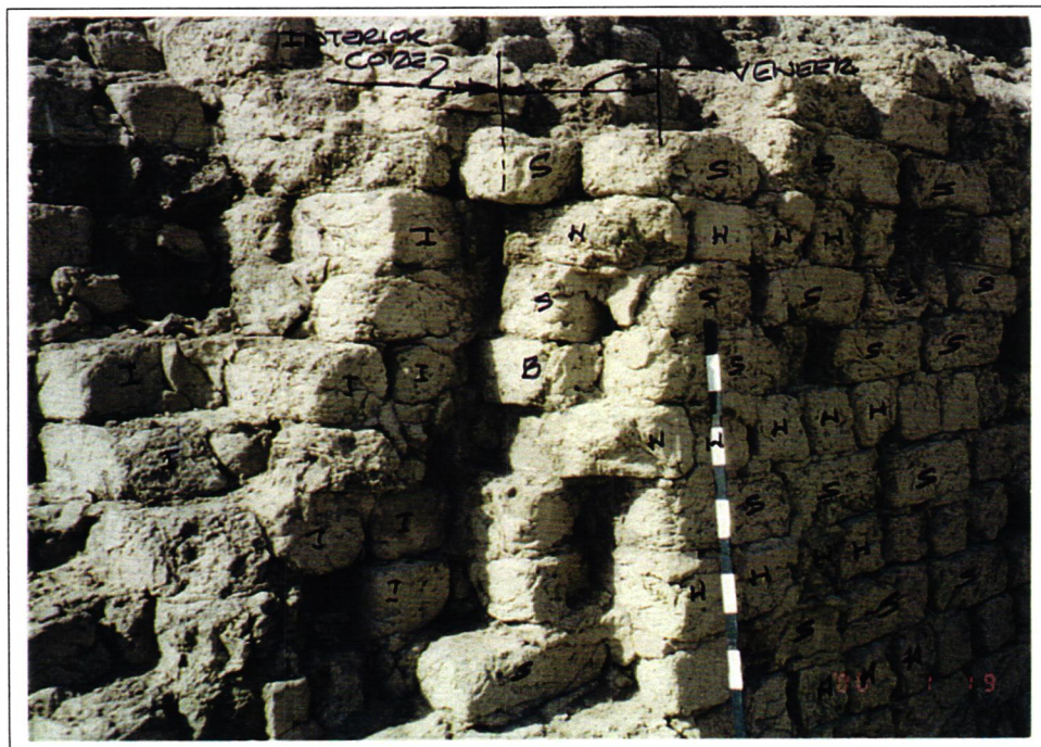
Photograph No. 6 Veneer Coursing
