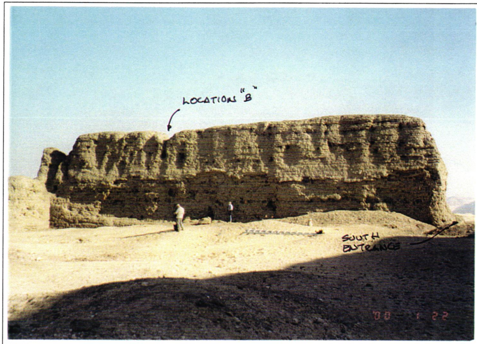
Photograph No. 119 South Main Enclosure Wall, Interior View
