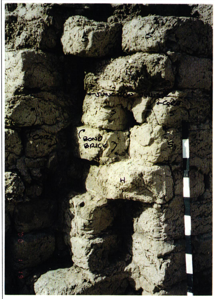
Photograph No. 7 Bond Bricks
