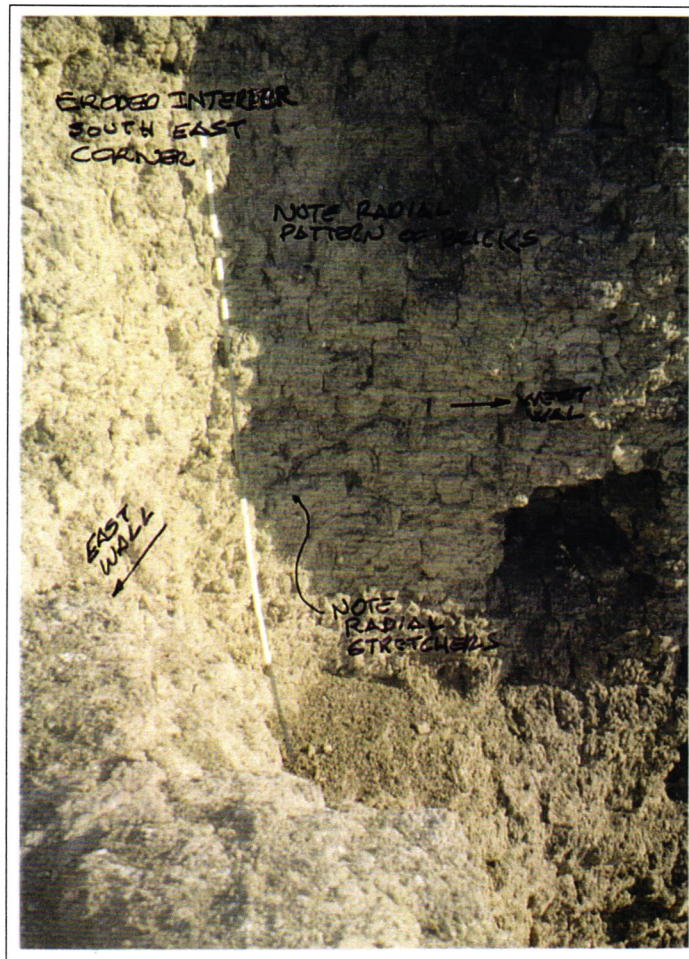
Photograph No. 17 Bonding at Main Enclosure Wall Corners
