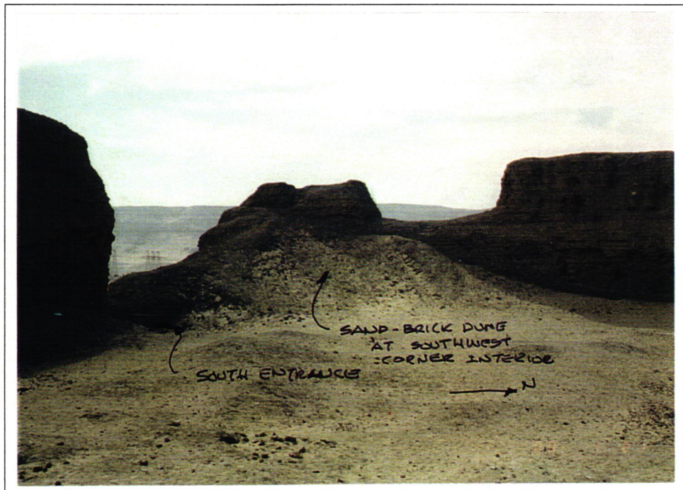
Photograph No. 118 South Main Enclosure Wall, Southwest View
