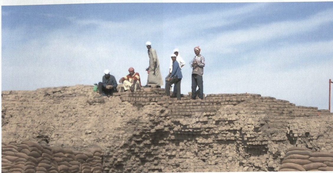
Figure 7: Capping the top of the east enclosure wall.
