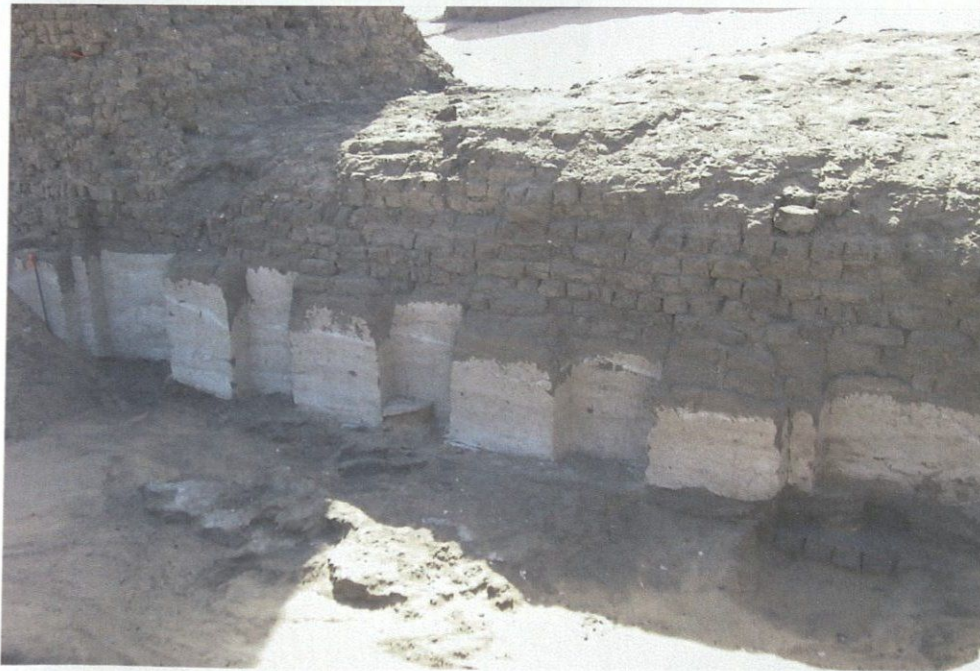
Figure 1: Plaster remains on the lower part of the east side of the East Enclosure Wall, near the north end.
