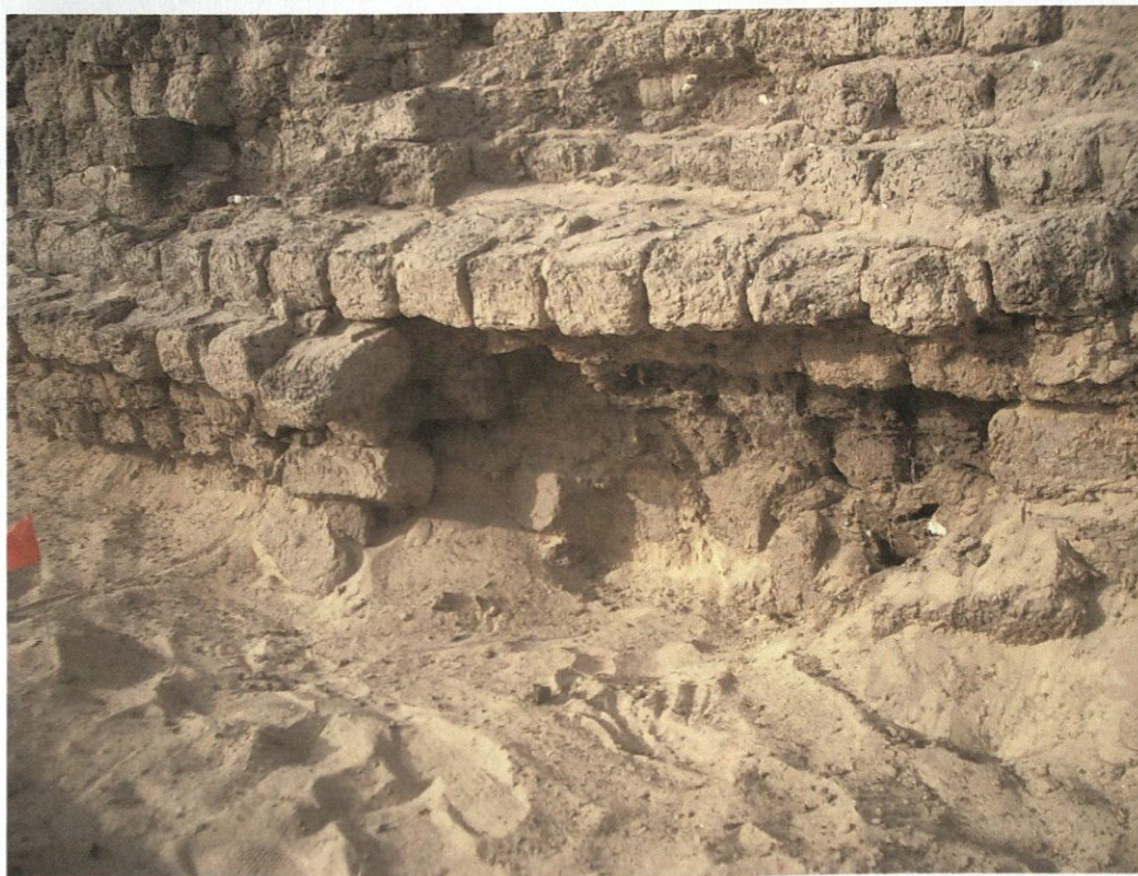
Figure 3: Unstable base of west enclosure wall, east side, along the south portion.
