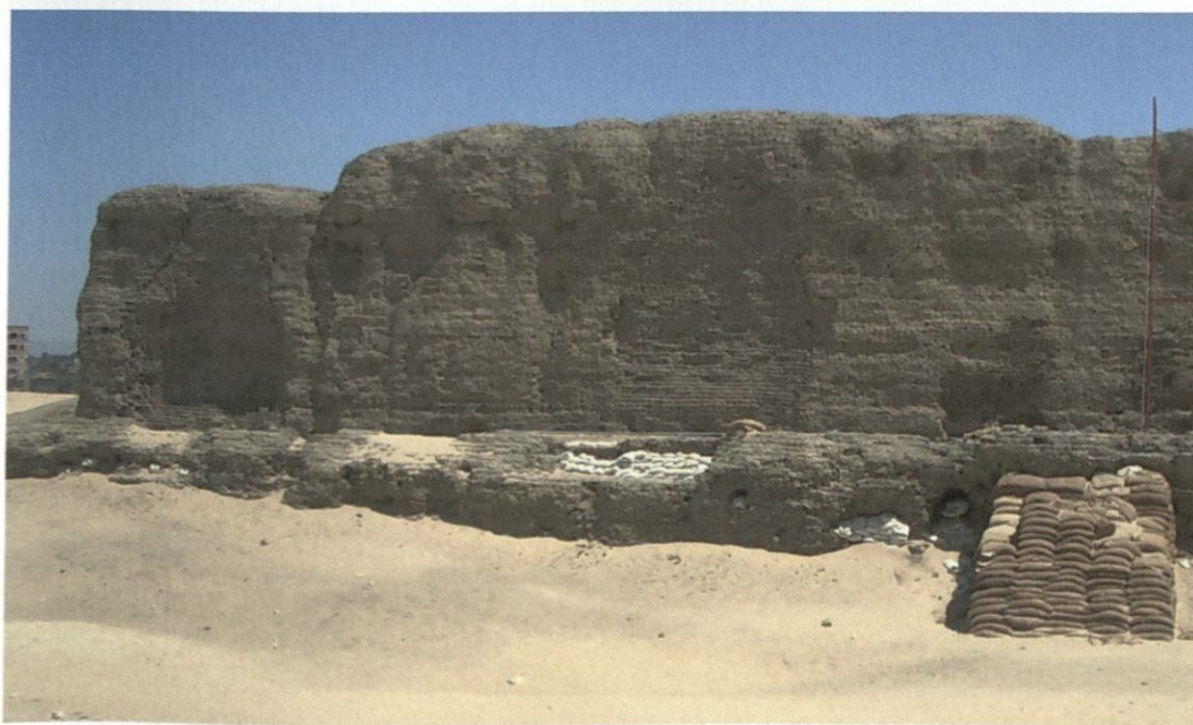
Figure 8: West wall with stabilized north Coptic cells with new masonry textured and washed
