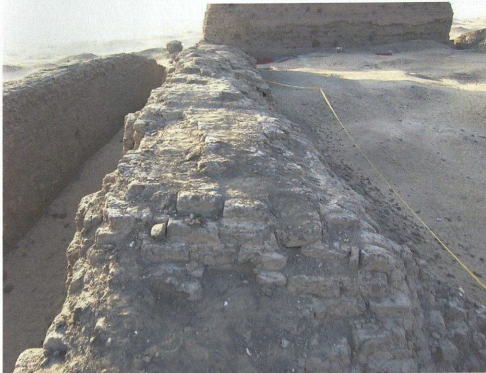
Figure 1: A section of the east enclosure wall with eroded mud bricks on the top of the wall.
