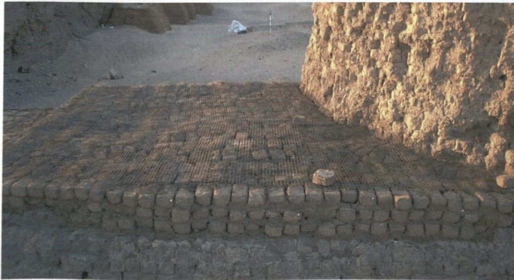
Figure 4: Geogrid horizontal reinforcement installed.
