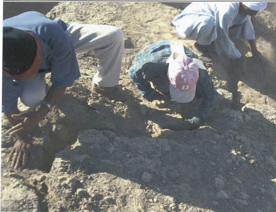
Figure 8: Crack on top of east wall being cleaned out
