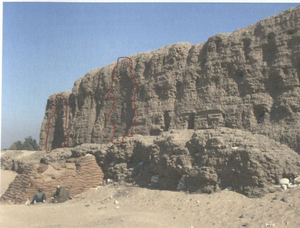
Figure 6: The character of the original walls is reflected in the stabilization of the north end of the west wall in the area where two large Coptic cells were stabilized. The reconstructed sections are outlined in red.
