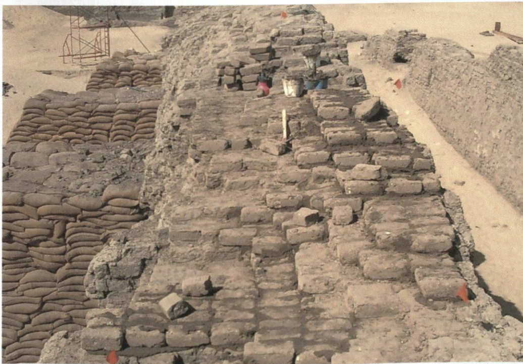
Figure 8: Capping while reflecting the general contours of the existing.
