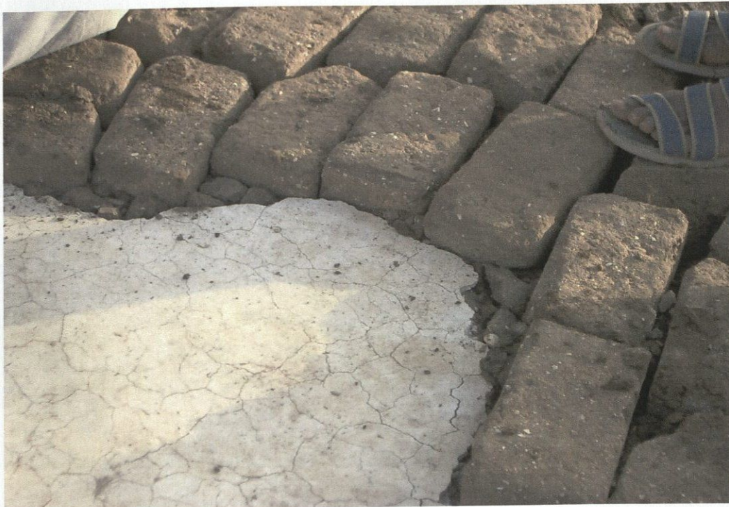
Figure 7: Mud brick has been raised to one course above cell floor.
