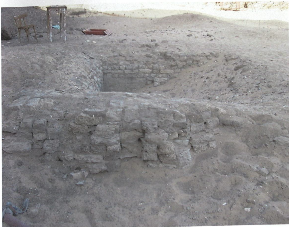
Figure 1: This area in the southeast corner of the Shunet should be backfilled, but until it is, the exposed mud brick walls should be protected with sandbags.
