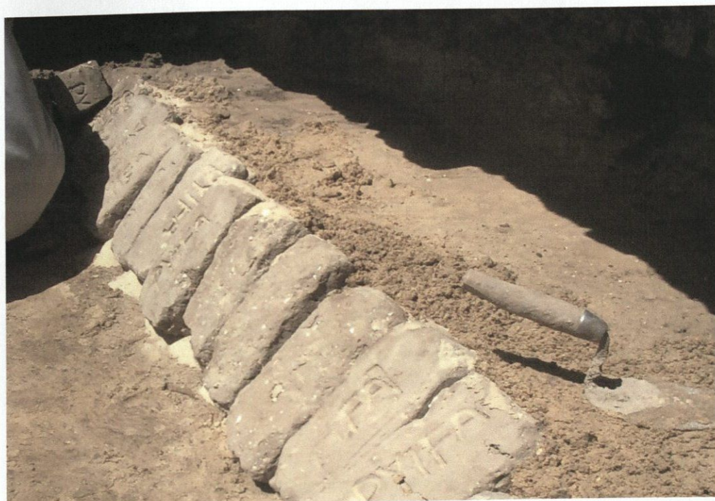
Figure 4: A separate feature has been constructed to retain the sand during compaction and placement of new mud bricks.
