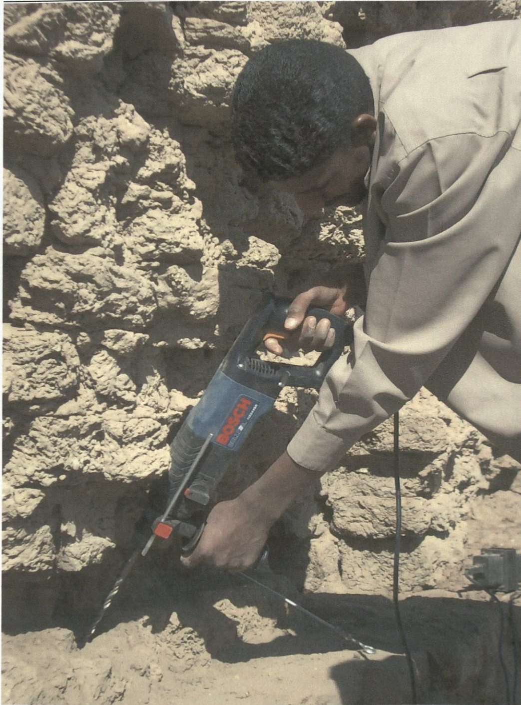
Figure 2: Holes are drilled at an angle of approximately 30-45% from horizontal.
