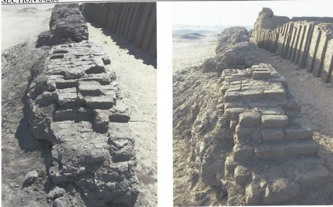
Figure 9: Another before and after comparison of the wall capping. The before on the left is after the wall was cleaned and debris and deteriorated mud bricks were removed.
