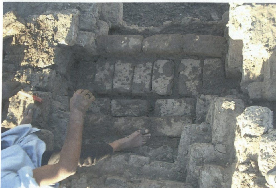
Figure 11: Mud brick is being laid over crack.
