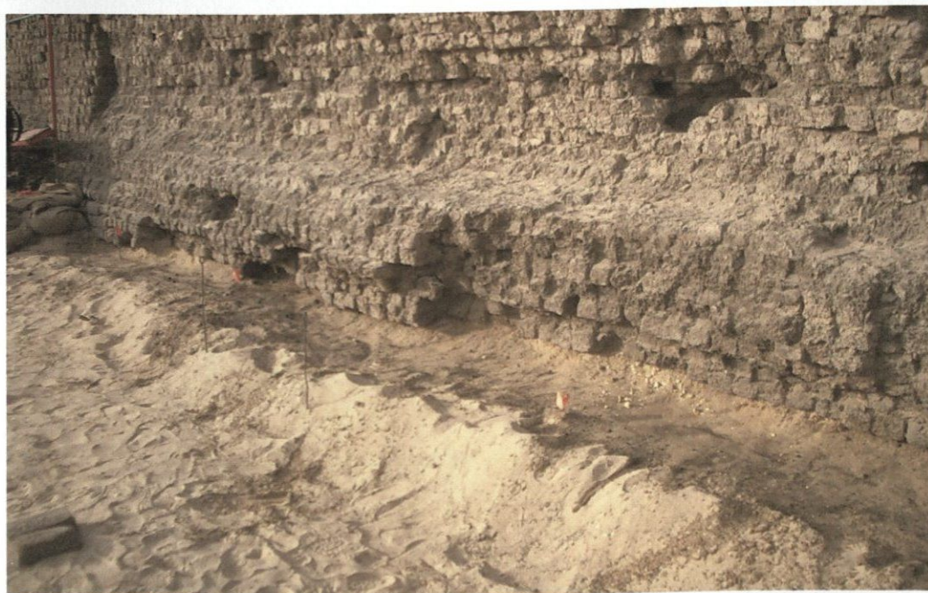
Figure 4: Loose materials have been removed and sand base is being compacted.
