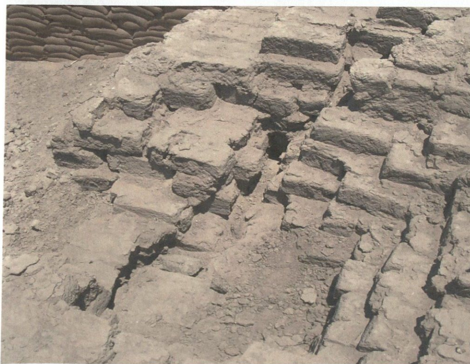
Figure 9: Crack shown in Figure 8 has been cleaned and loose bricks and materials removed.
