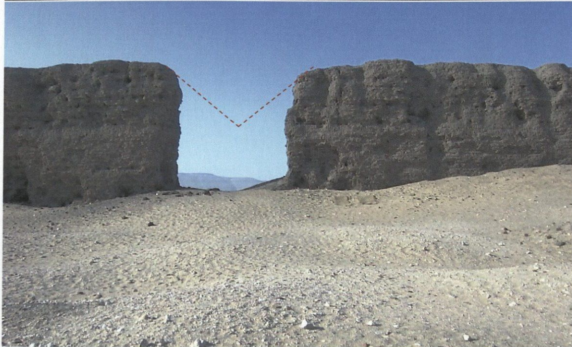
Figure 1: The west doorway prior to beginning the structural stabilization and partial restoration. The dashed red lines indicate the approximate extent of the mud brick construction necessary to establish structural integrity.
