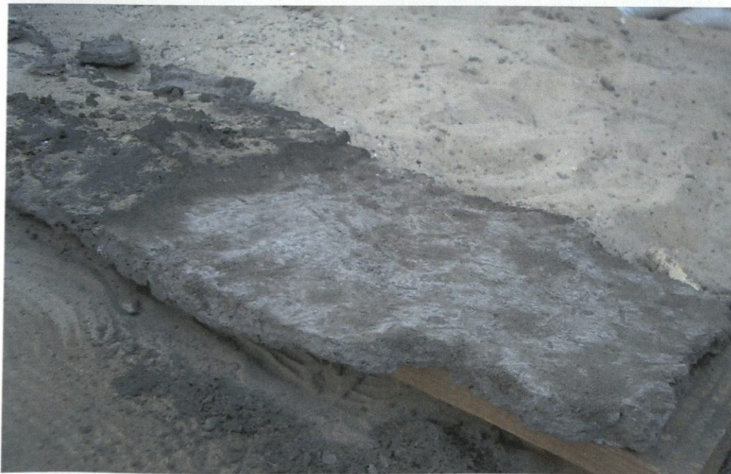
Figure 5: Large piece of plaster with partial removal of the mud plaster substrate.
