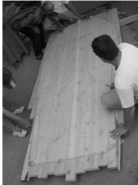
Fig. 2. Timbers for platform module assembled, with tracing of lid outline.
