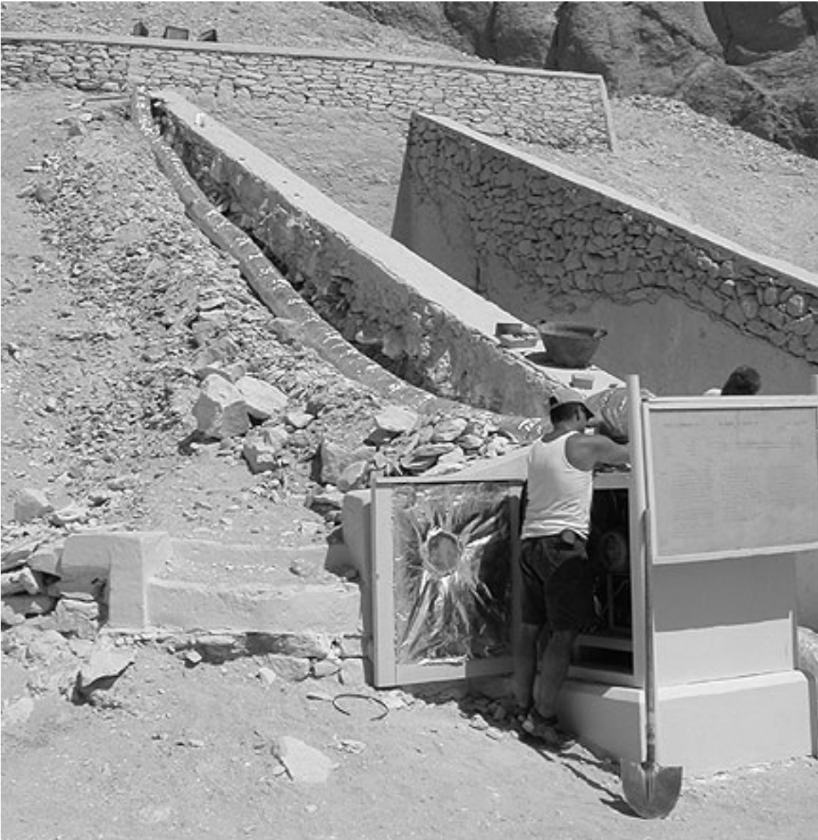
Figure 1. Exhaust tubing set into trench.
