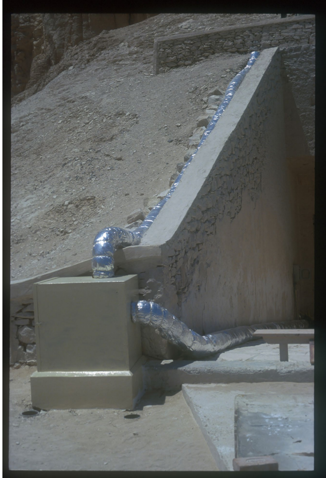
Fig. 5. Painted wooden housing for the exhaust fan with flexible tubing connected.
