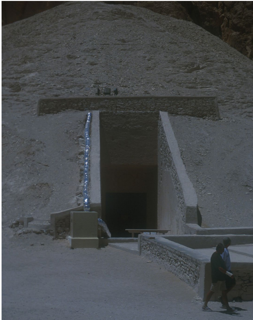
Fig. 6. Exhaust fan housing and foil-covered flexible tubing outside KV 9.
