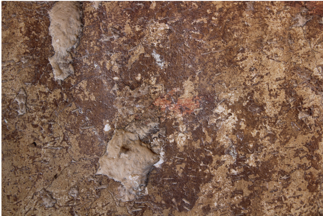
Detail, build up of surface deposits
