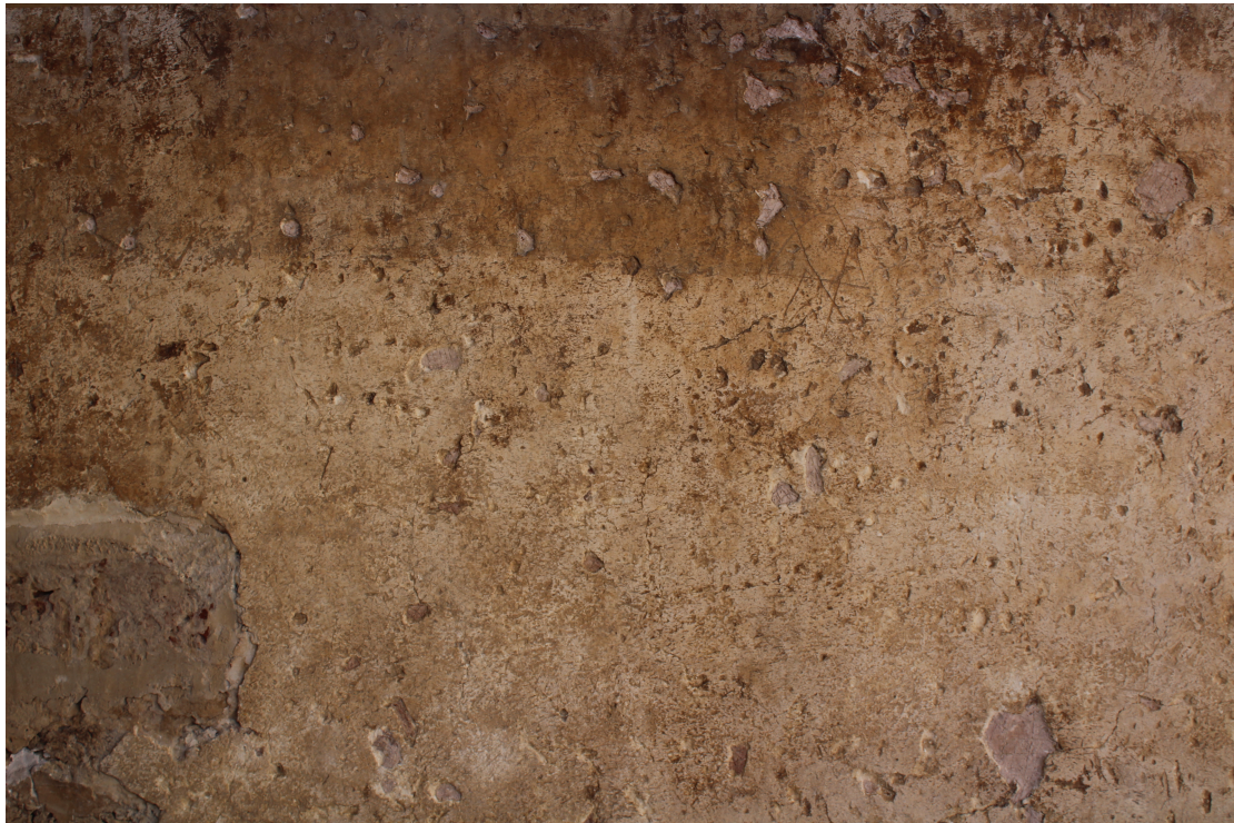
The plaster during the cleaning process
