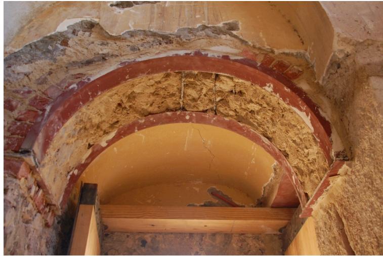
Supporting steel frames during installation
