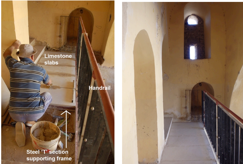
The mezzanine balcony during (left) and after (right) works
