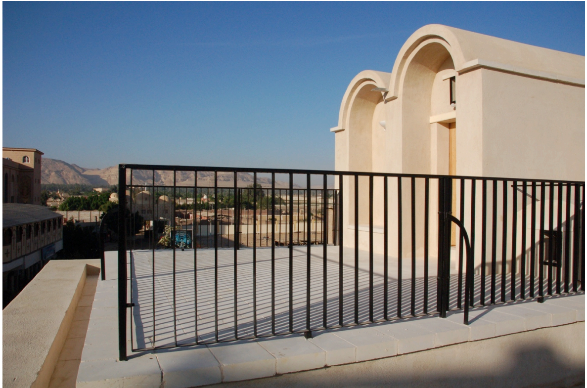
View of new roof terrace from the southeast
