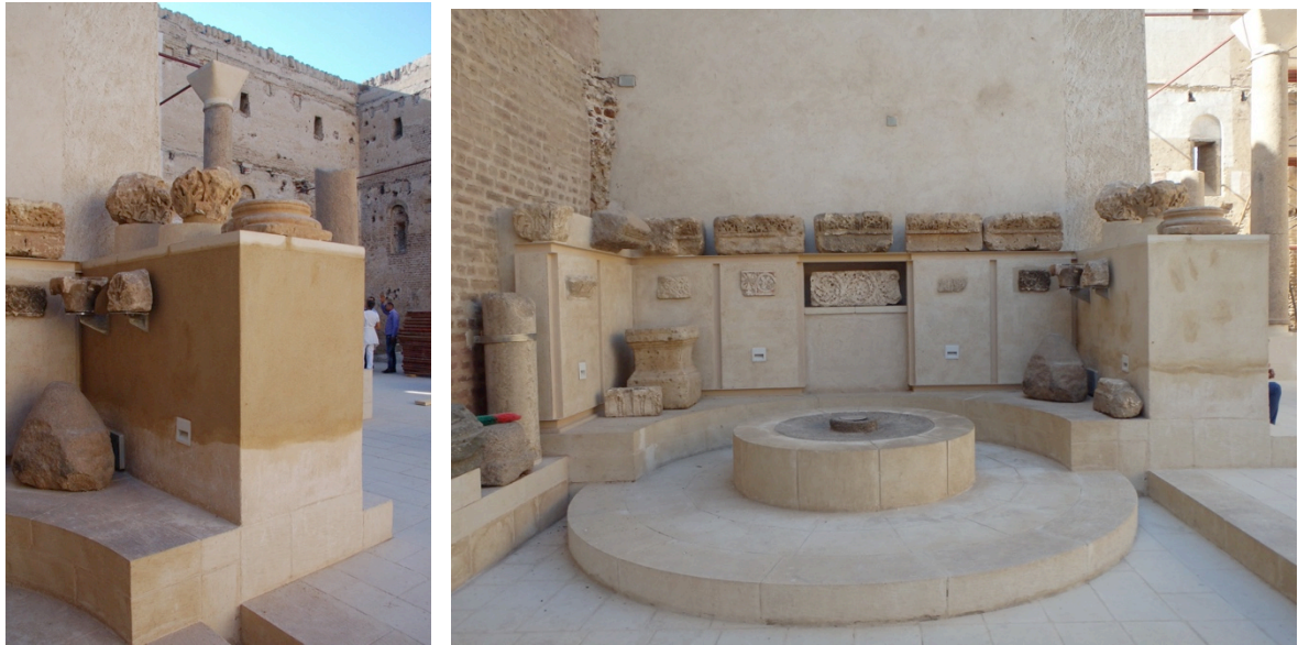
New section of lapidarium under construction (left) and completed additions to lapidarium (right)
