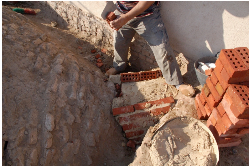
Construction of relieving arch over corner pendentive of a dome
