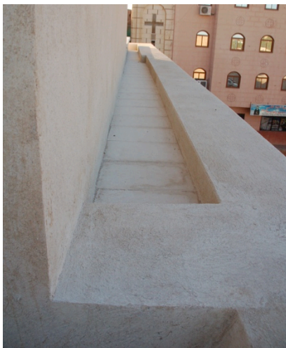
Stone lined drainage channel on west side of roof (left) and entrance to terrace from staircase (right)
