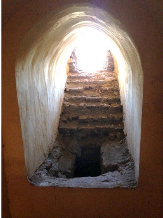
View of the location of the brick shaft in the high-level window embrasure at the east end of the east-west ground floor corridor (note limestone slab covering).
