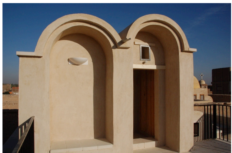
Stone lined drainage channel on west side of roof (left) and entrance to terrace from staircase (right)
