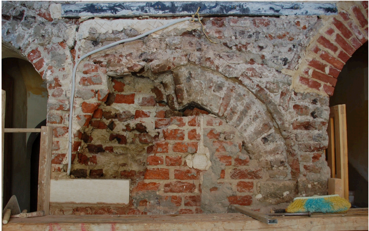
Arch over blocked opening to well during reconstruction of missing section
