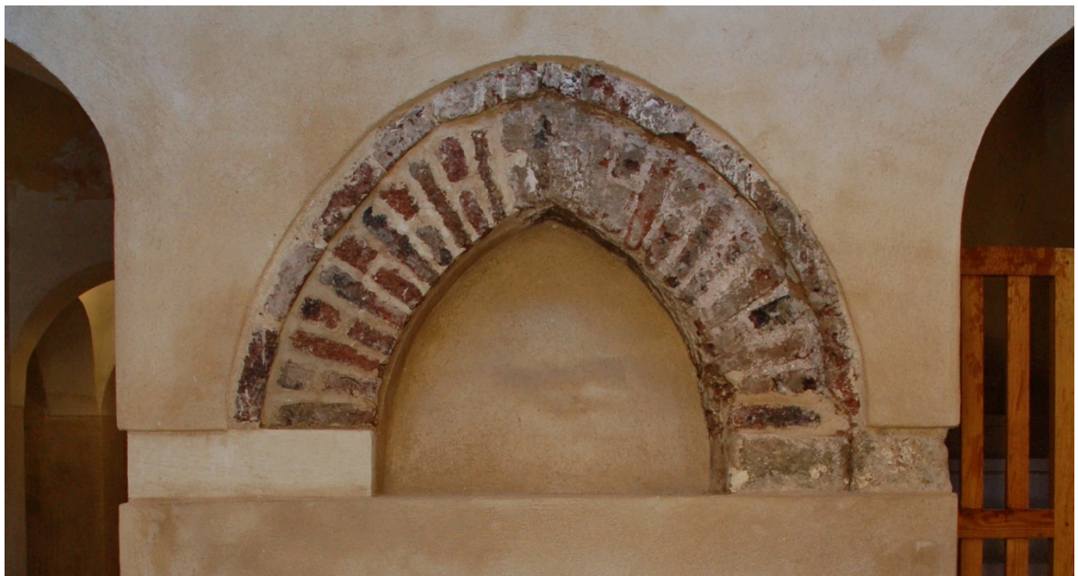
Arch over blocked opening to well after reconstruction of missing section
