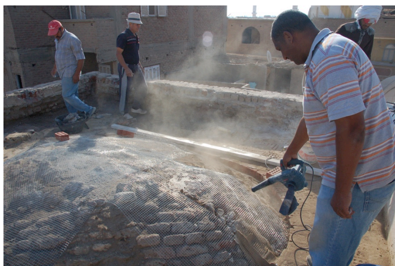
Cleaning surfaces of the vaults
