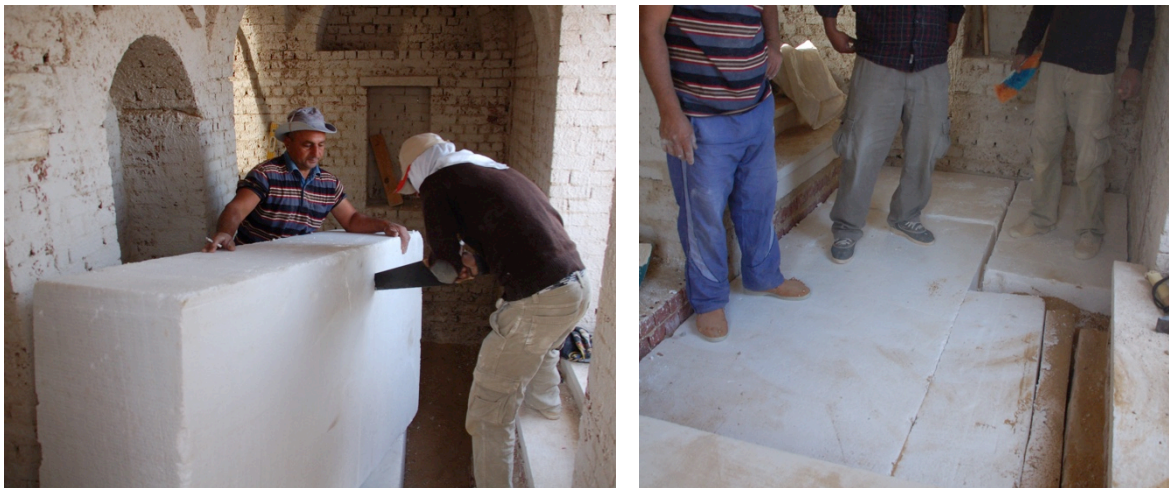
Installation of white foam block on stair landing to reduce loading
