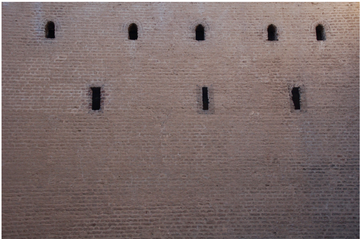
Fenestration of the east wall of the tower after intervention
