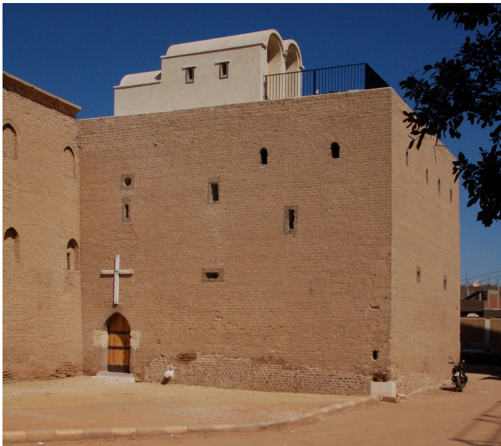
Views of the new staircase structure from the north (top left), east (top right) and west (bottom)
