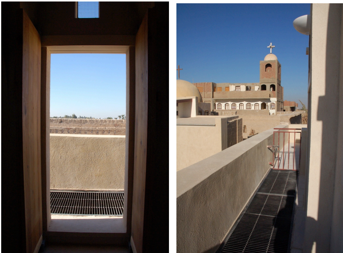
Approach to the viewing deck (left) and the steel grille viewing deck with gate to eastern side of roof (right)
