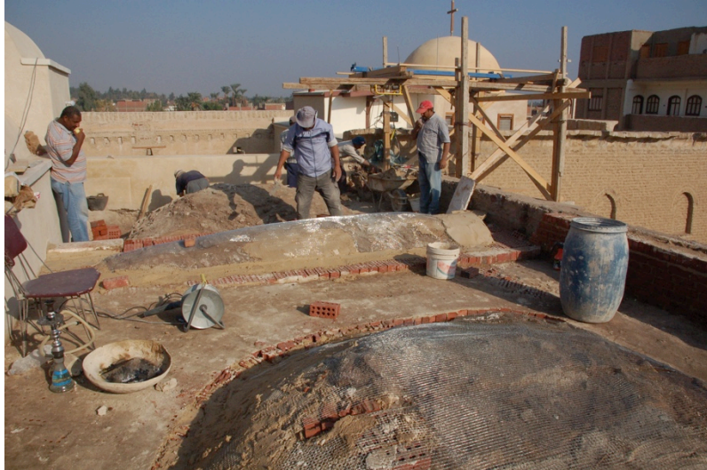
Covering the exposed areas with galvanised mesh
