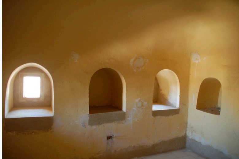
Treatment of windows and niches on first floor
