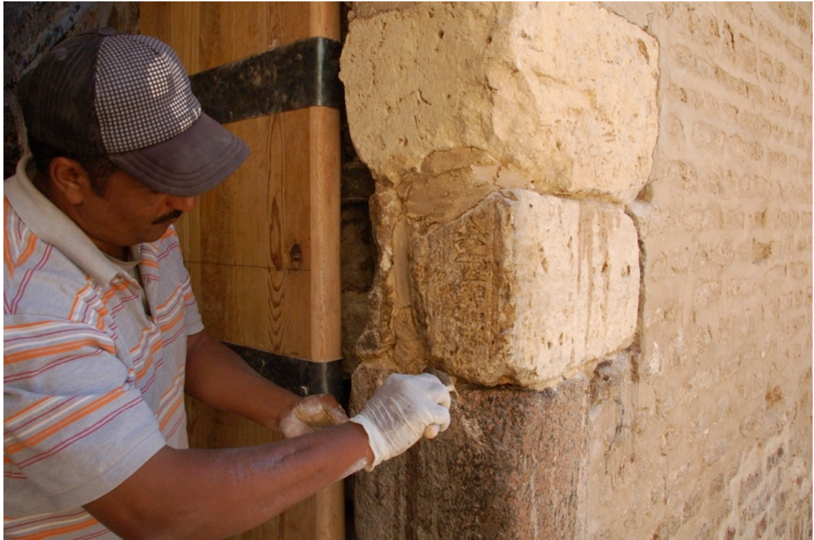
Conservator Hani al-Taiyyib pointing the block with hieroglyphic inscription in the entrance door to the tower after cleaning with dilute ammonium carbonate poultices
