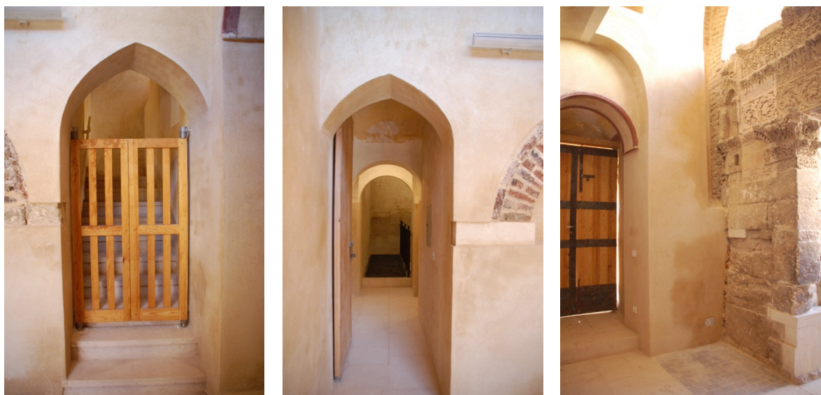
Wooden grille gates on staircase (left), door to inner rooms (center) and back of entrance doors (right)
