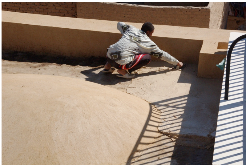
Plastering the domes and roof surface
