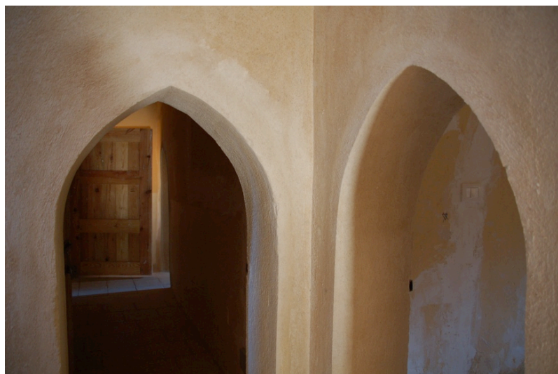
The doors to the first floor after finishing works
