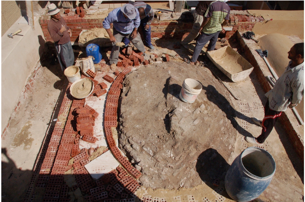
View from west of cantilevered stone slabs and brickwork on north side of north dome
