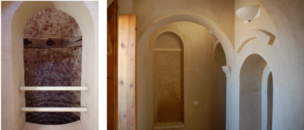
Opening to the well with pulley block emplacement (left) and general view of upper landing with opening to well at right, and blocked access door to terrace in background (right)
