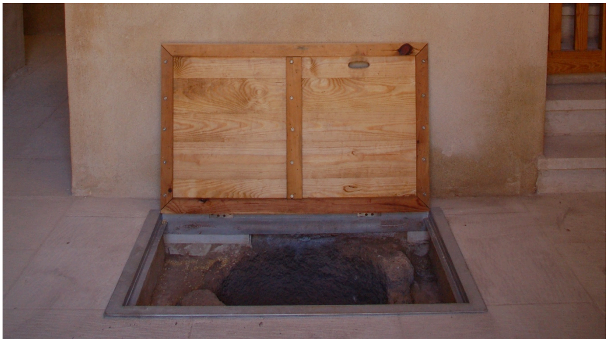
Detail of trapdoor over basin in entrance area
