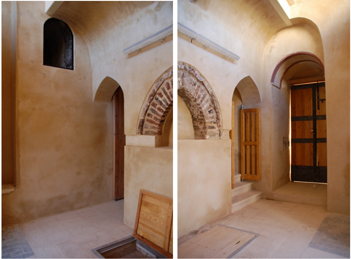
General views of entrance area after treatment
