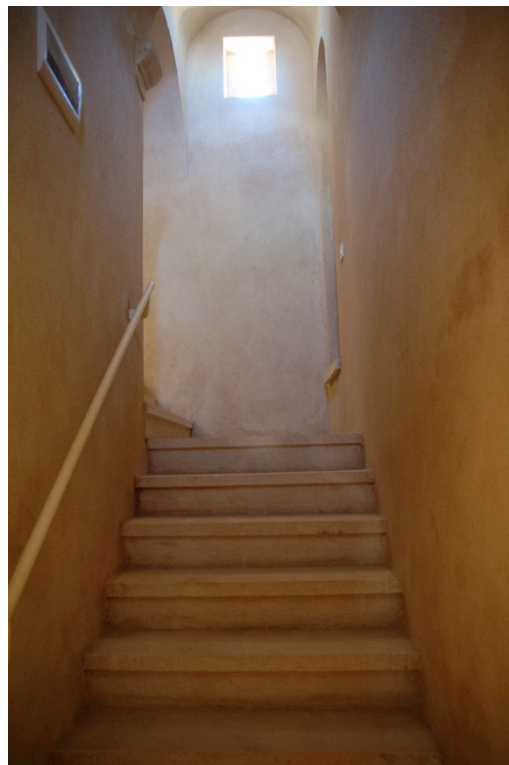
General view of staircase leading to viewing deck from first floor
