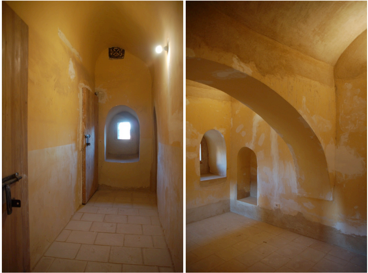
General views of first floor corridor (left) and west room (right) after works
