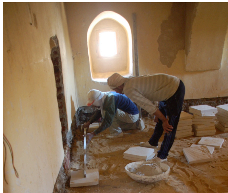
Tiling in progress on first floor
