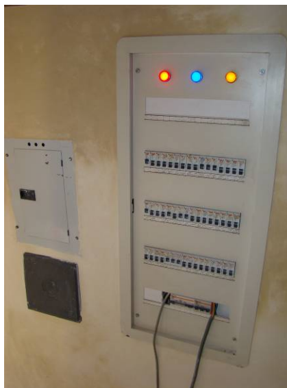
Main electric panel installed in the staircase entrance
