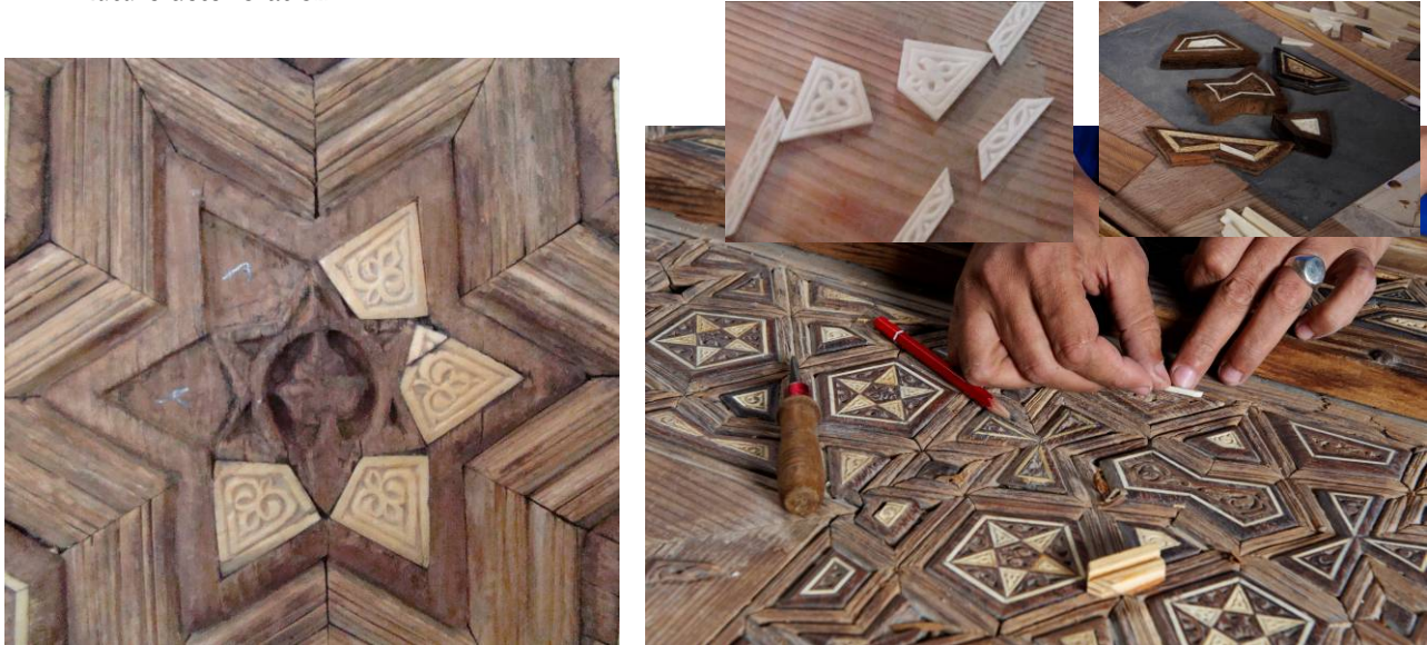
Restoration work on inlaid wooden doors; missing pieces replaced by carved camel bones
