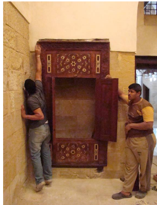
Installation of inlaid cupboards
