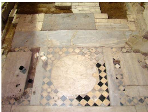
View of the marble replacement in the courtyard
