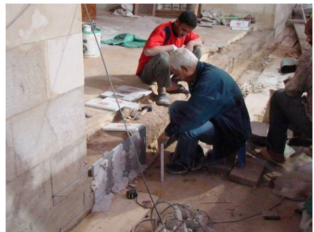
Installation of the marble panels on the Qibla step
