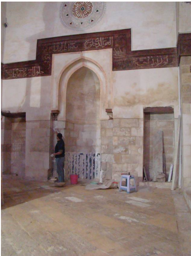
Stone conservation and re-pointing of joints
