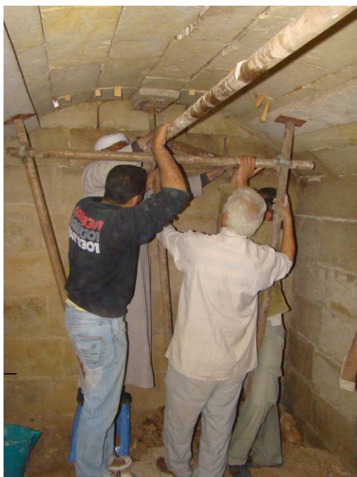
Structural consolidation of the vault
