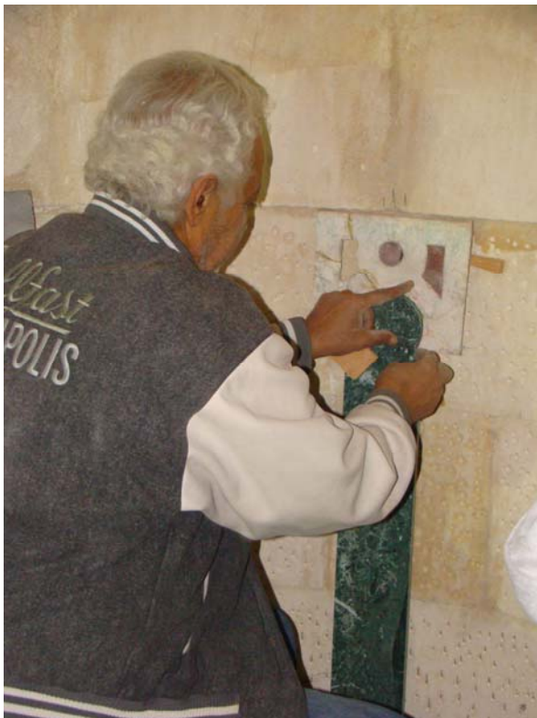
Installing the old marble panels in the mihrab
