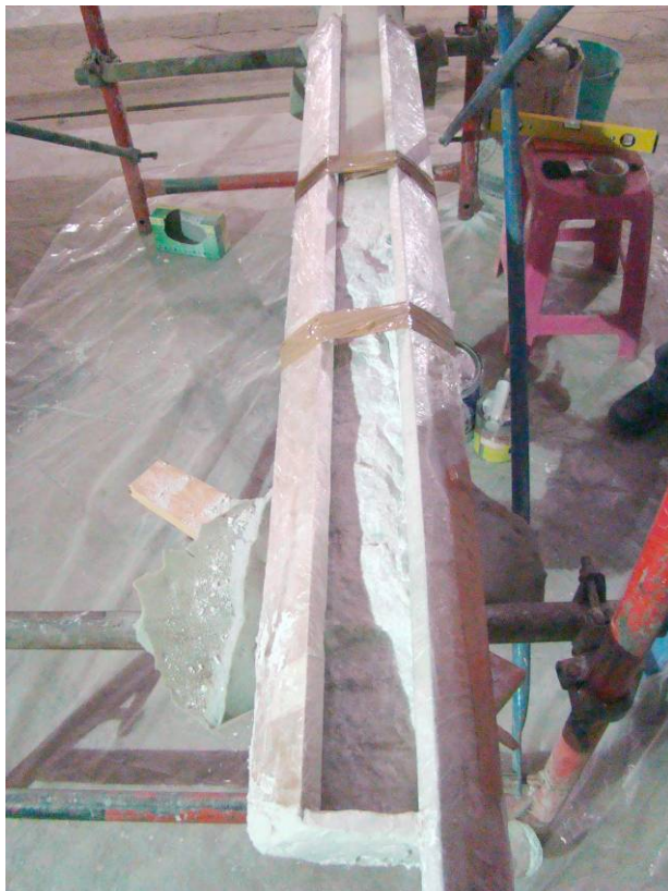
View of the cast surrounding the column
