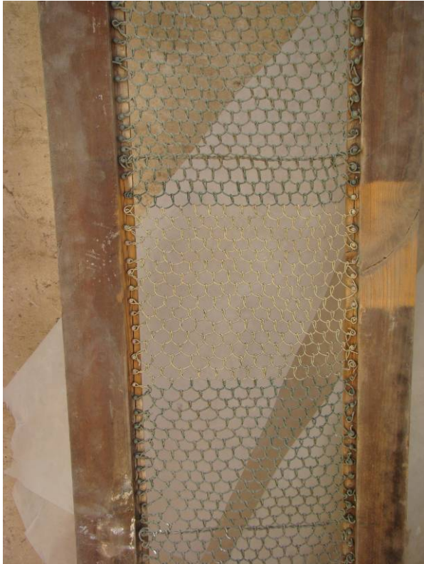
Cleaning and completion of the missing mesh parts of the façade windows
