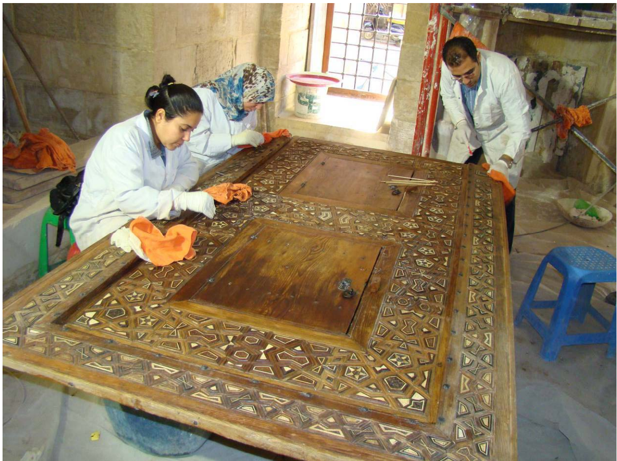
Applying micro-crystalline wax protection
