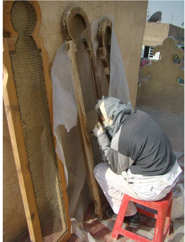
Cleaning and completion of the missing mesh parts of the façade windows
