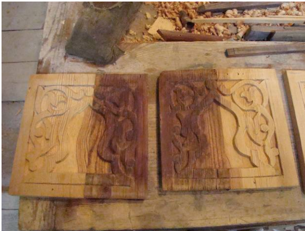
Restoration of the missing parts of the wooden panels
