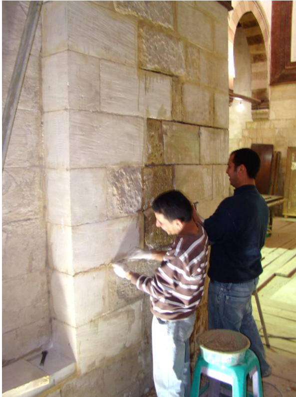
Re-pointing of joints in the western iwan
