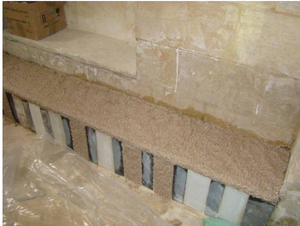
Cleaning of the marble tiles by poultices
