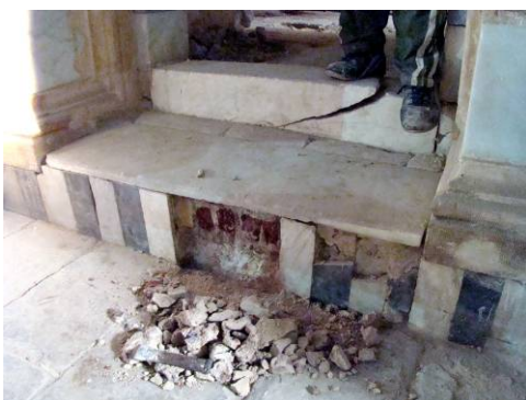
Cleaning of the stone and marble tiles
