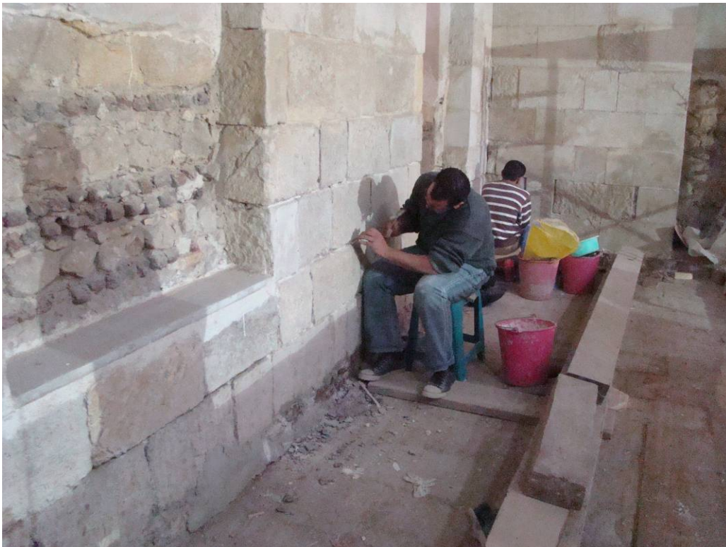
Cleaning of stone courses and re-pointing of joints
