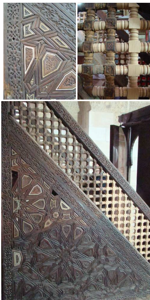
New turned wood replacing missing parts
