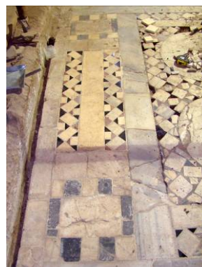
View of the marble replacement in the courtyard
