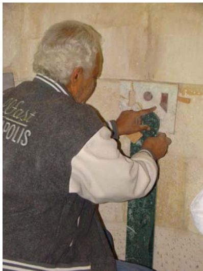
Installing the marble panels
