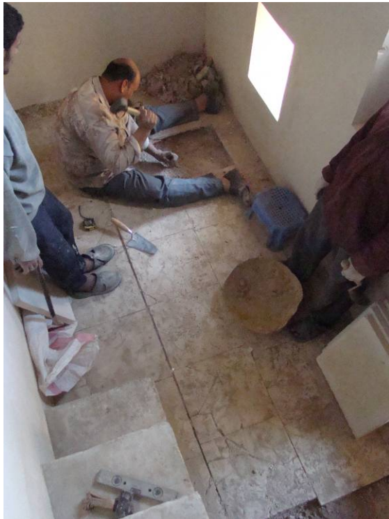
Stone tiling replacement in M2
