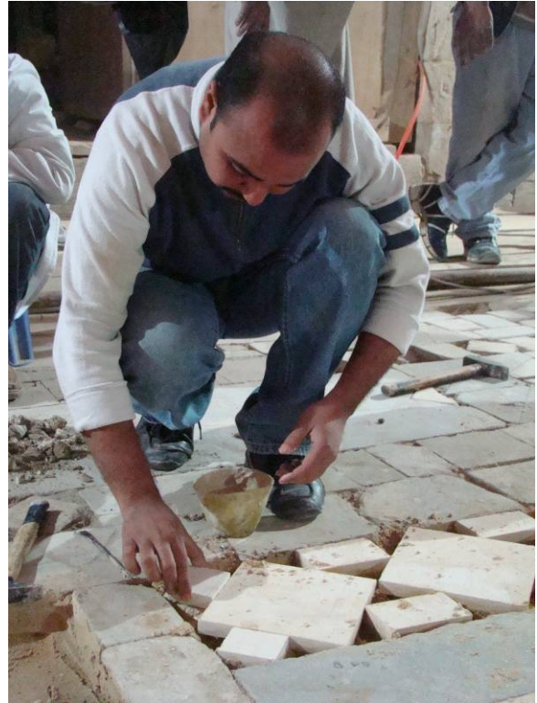
General view of the marble tiling in the courtyard during conservation
