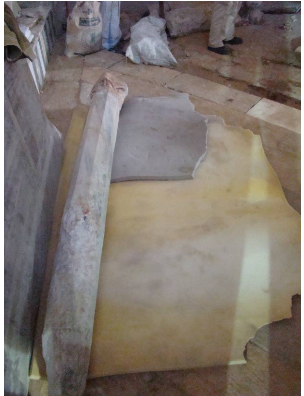
View of the badly eroded lower section of the column
