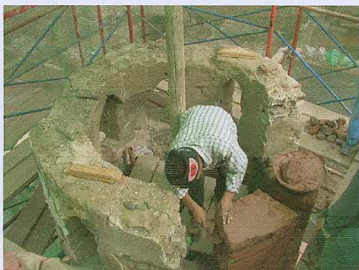
Reconstruction of the brick body
