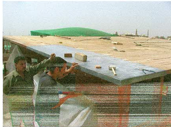
Installation of led sheets protecting the wooden ceiling
