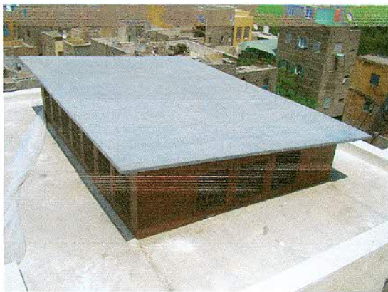
Restoration and painting of the wooden lantern
