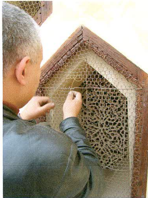
Restoration of the dome crescent and the copper mesh windows
