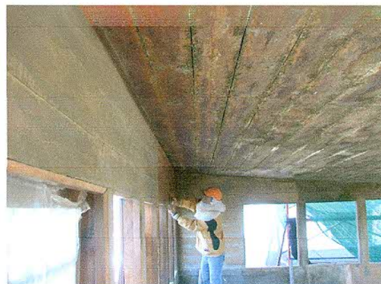
Installation of led sheets protecting the wooden ceiling
