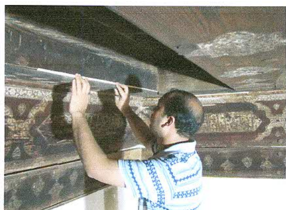
cleaning and consolidation of the wooden ceiling and inscription bands
