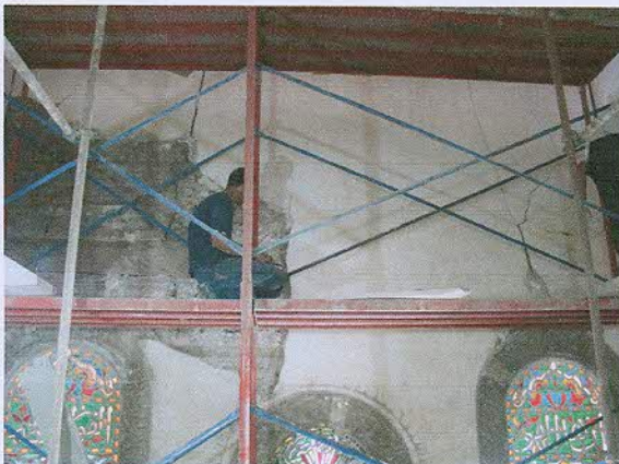
Removing and fixing detached original plaster layers
