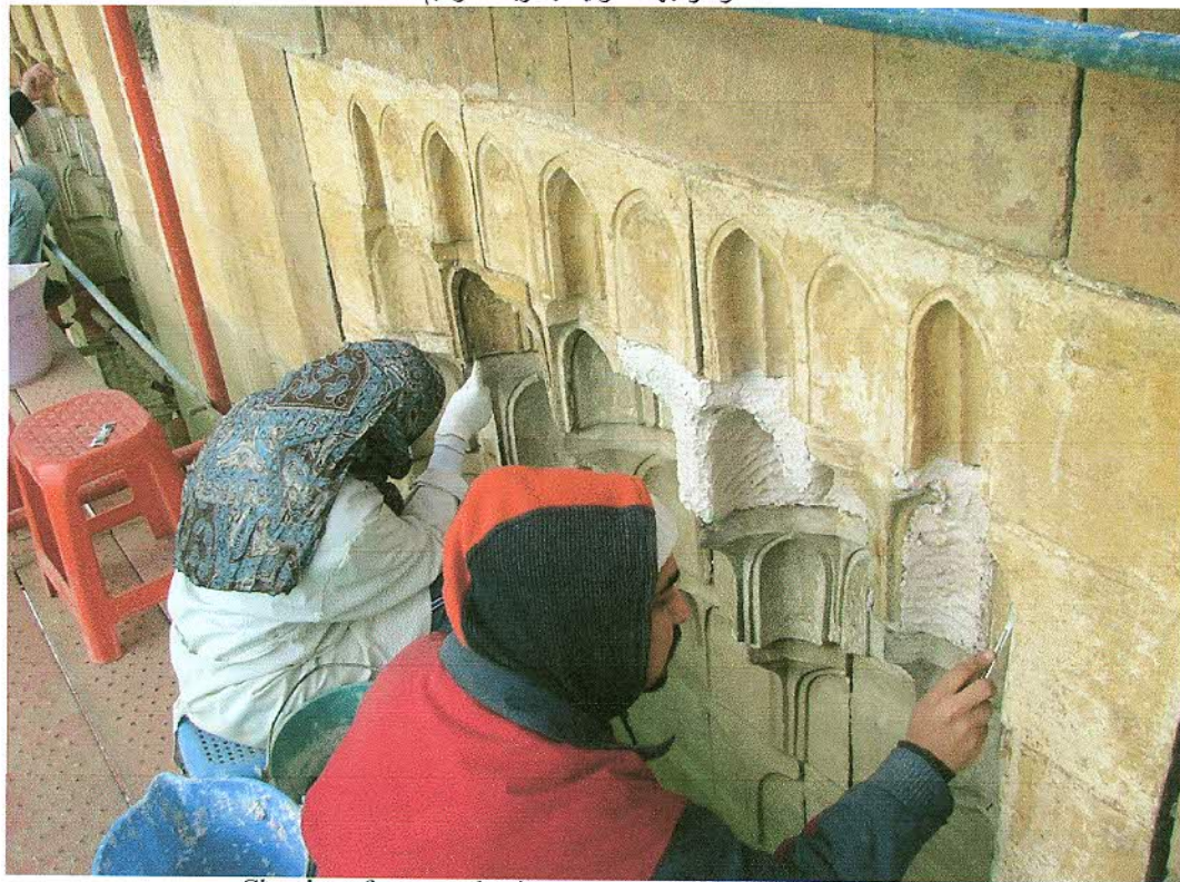
Cleaning of stone stalactites on the eastern façade by poultices
