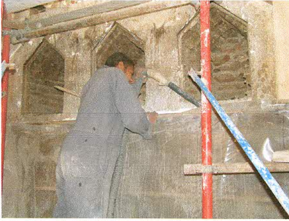
Cleaning and completion of the interior gypsum windows
