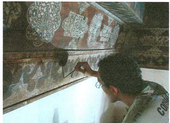
cleaning and consolidation of the wooden ceiling and inscription bands
