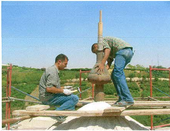
Restoration of the dome crescent and the copper mesh windows
