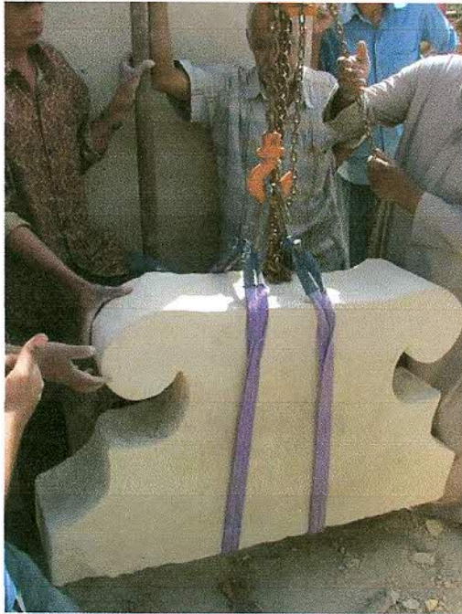
Cleaning and reconstruction of the lost stone crenellations
