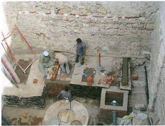
Reconstruction of foundations
