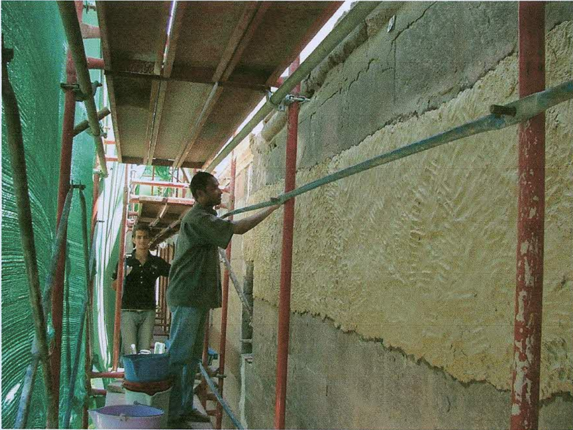
Chemical Stone cleaning with paper poultices
