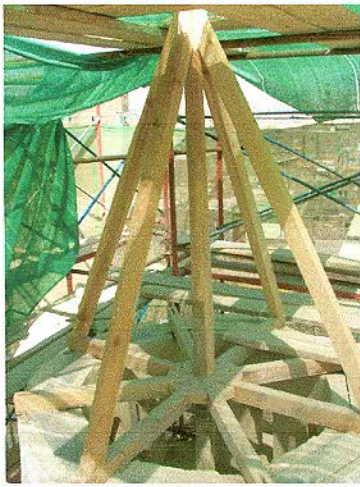
Reconstruction of the wooden cone and led installation
