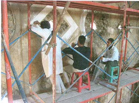
Cleaning the courtyard plaster layers
