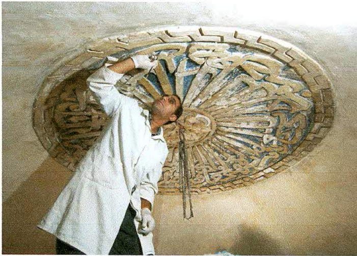
Cleaning of the stucco decoration in the top interior of the dome
