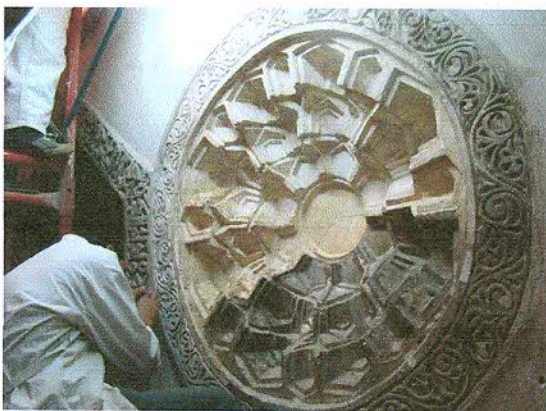
Cleaning the courtyard plaster layers
