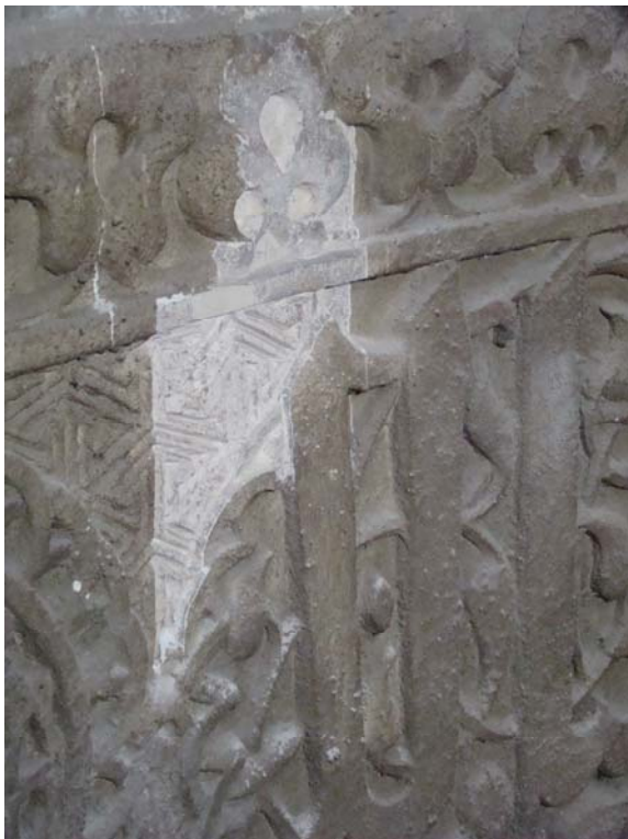
Different views of the inscription band covered with a hard crust of limewash and dust
