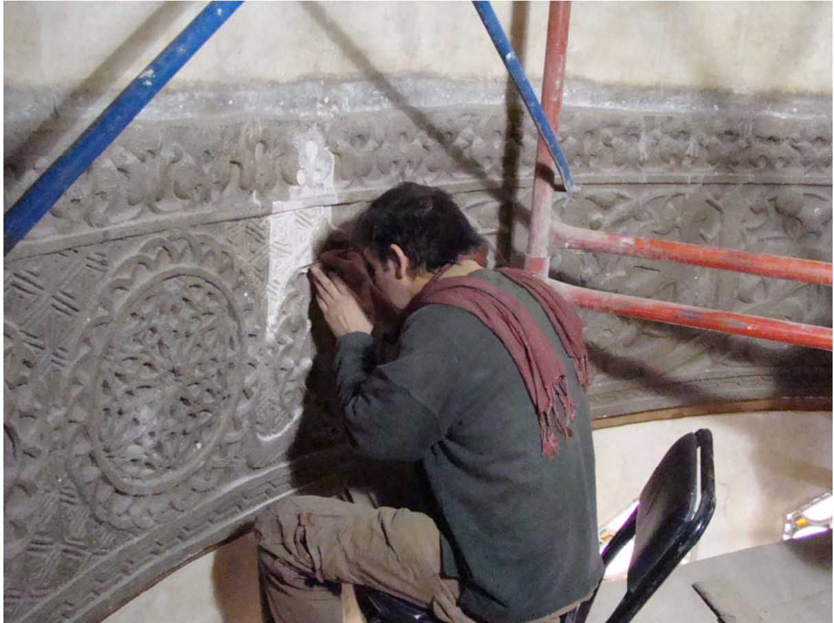
The conservator, Erico Peintner, carrying out cleaning tests of the inscription band
