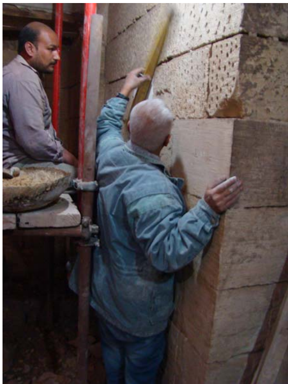
Stone replacement activities in the lower part of the dome
