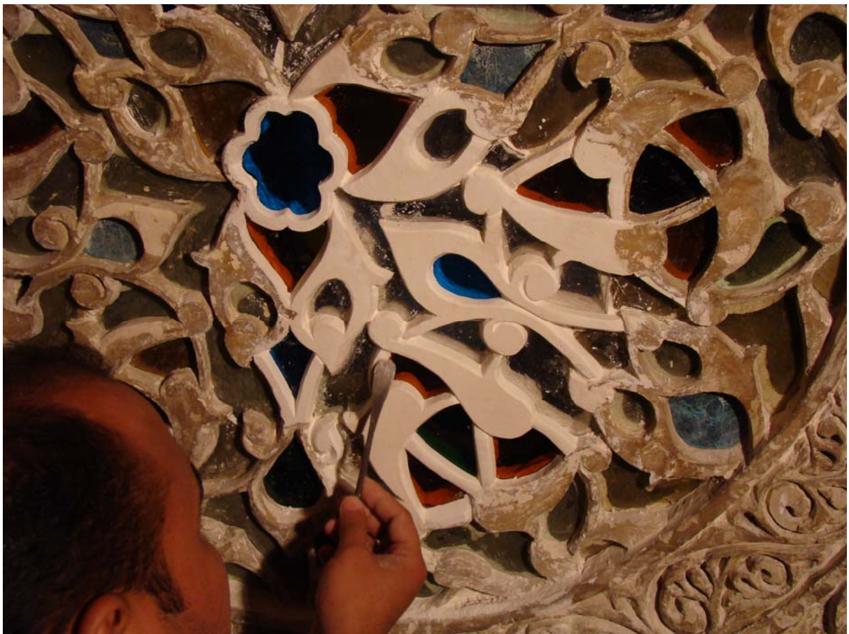
Completing the missing (and lost) parts of the stucco decoration in the west iwan
