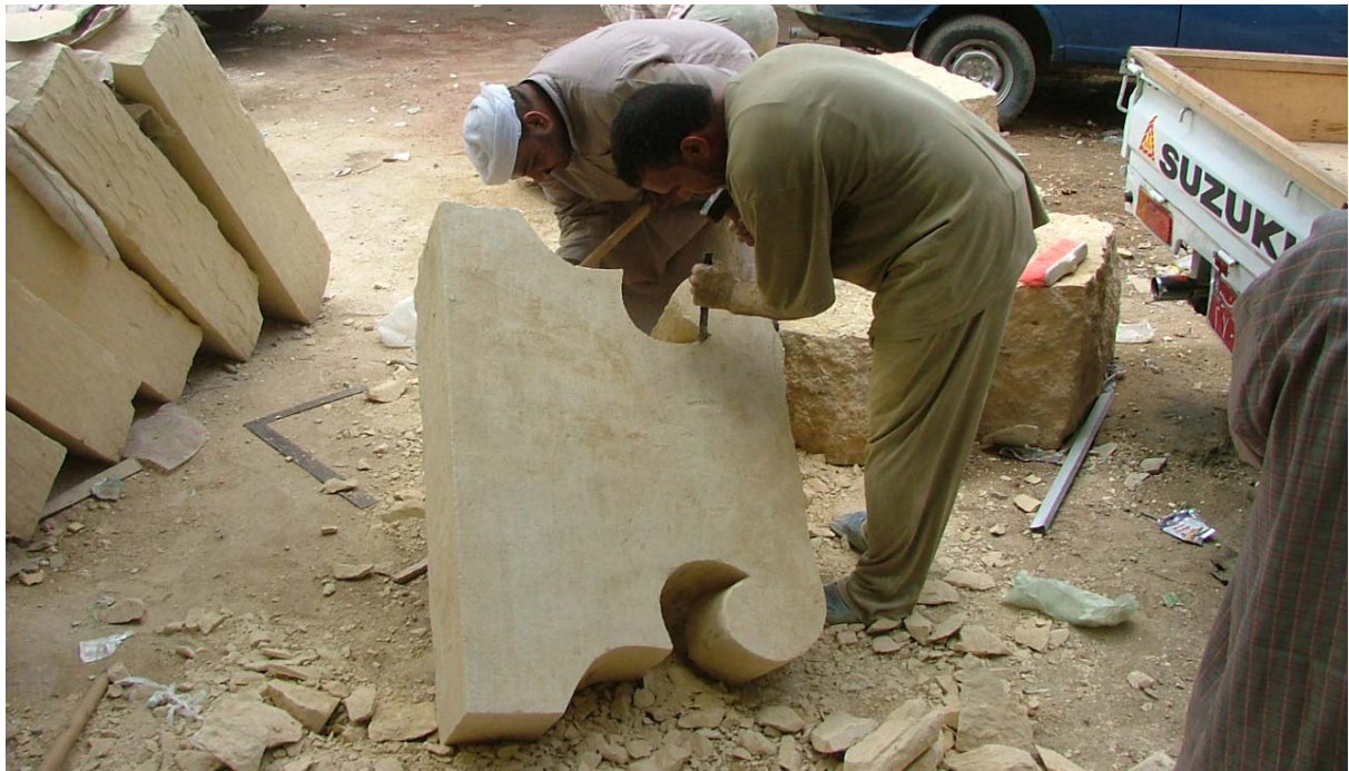
Carving the missing crenellation of the south (main) façade
