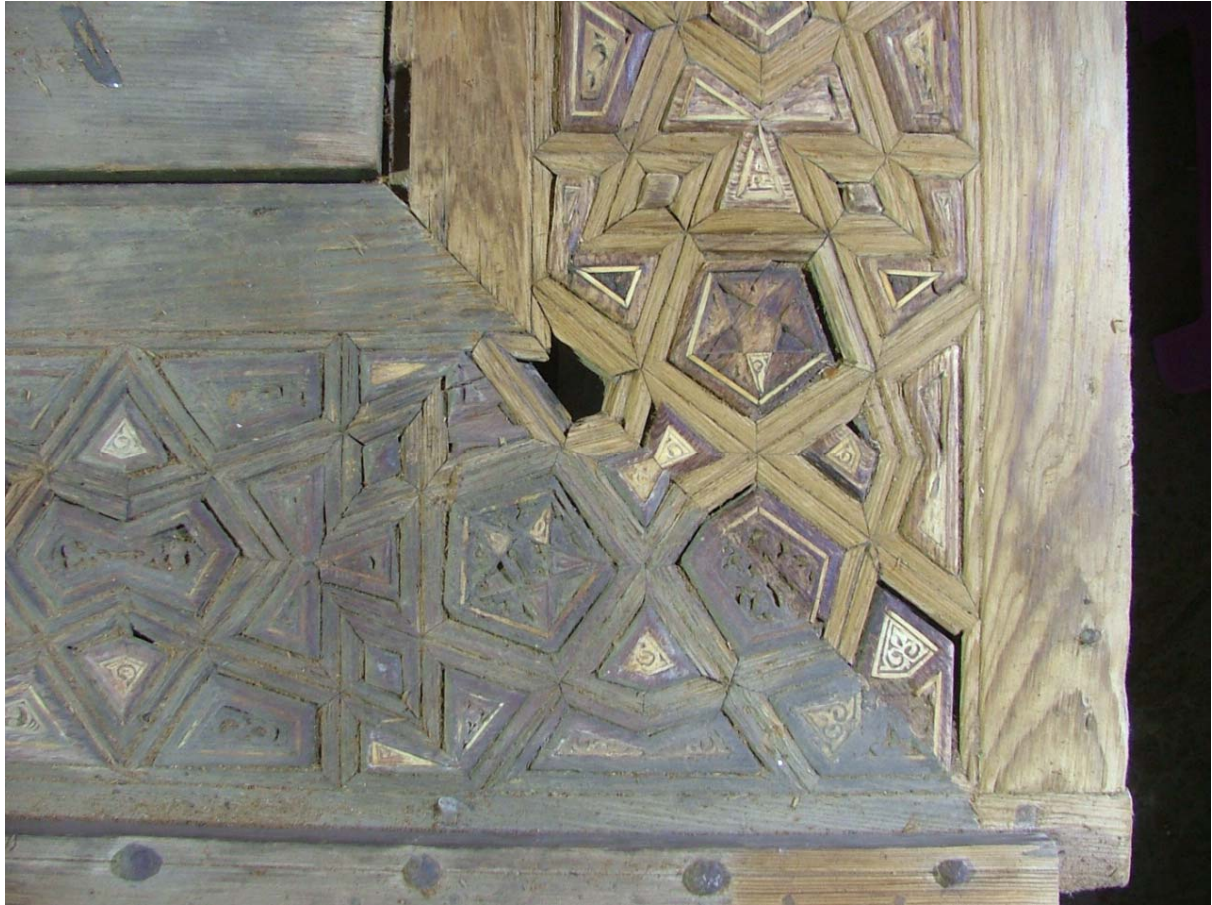
Sample of cleaning the wooden shutters of the niches of the qibla ivan
