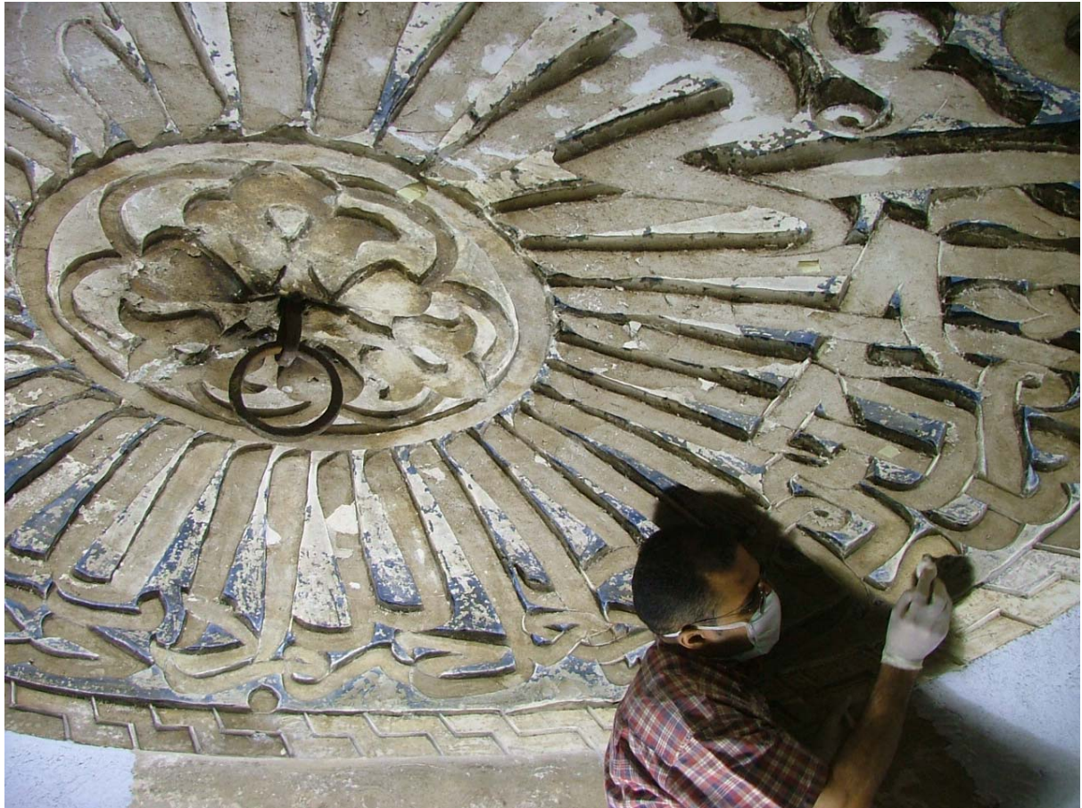
View of the roundel during cleaning
