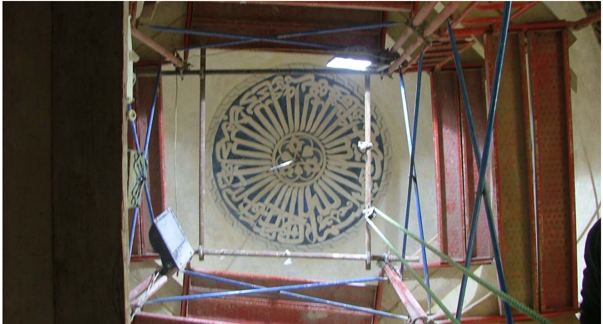
View of the upper roundel after cleaning and retouching the blue background; below: detail of the roundel
