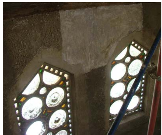
Activities and details of removing the dust and the recent limewash layer around the first level windows of the mausoleum
