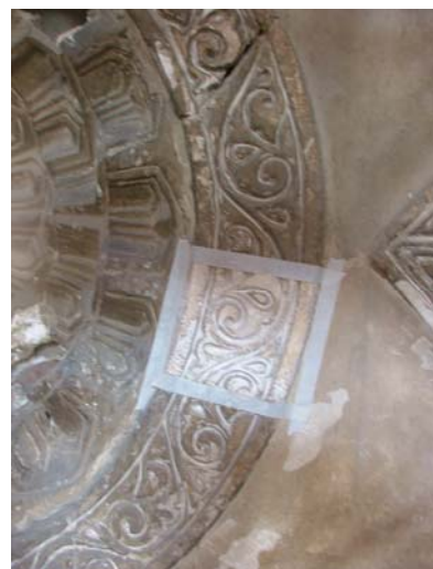
Samples of cleaning the gypsum mortar with poultice and with mechanical cleaning
