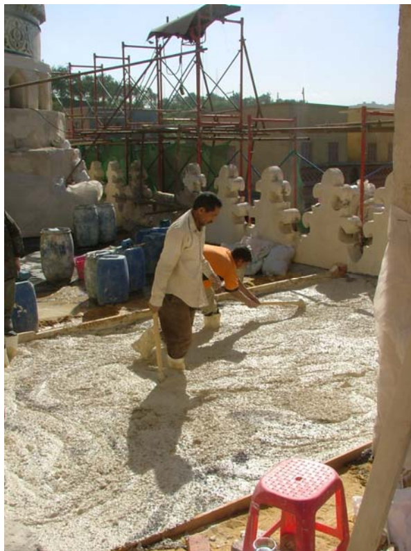
The upper insulation layer during application and after hardening
