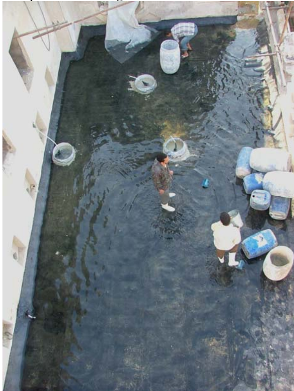
Insulation activities on the south ceiling and water testing the insulation before applying the upper mortar mix layer
