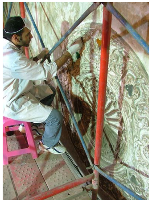
Activities of removing the fine dust from the decorated gypsum roundel in the qibla iwan
