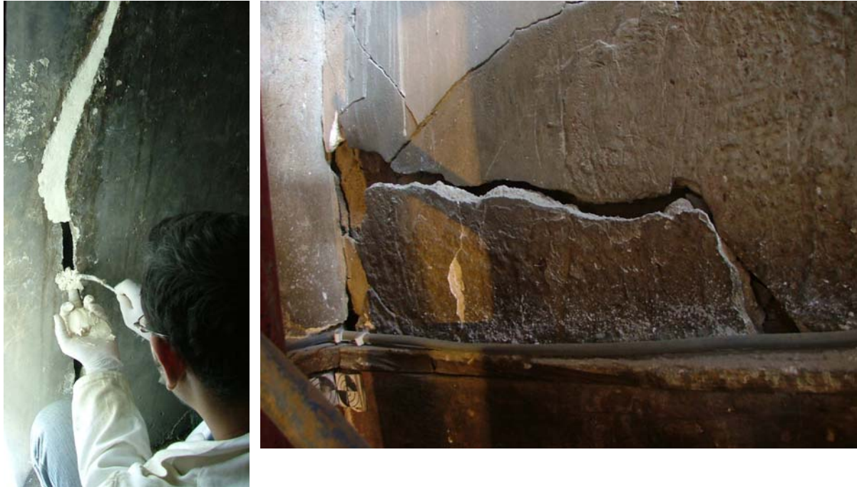
Example of the condition of the gypsum plaster in the courtyard showing serious cracks and detachment
