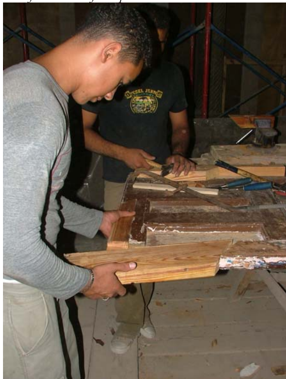
Architectural repair of damaged parts in the wooden shutters
