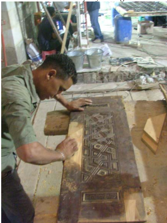
Architectural repair of damaged parts in the wooden shutters
