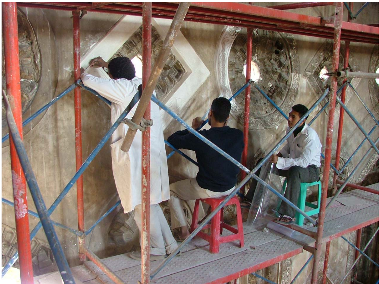
Activities of completing the gypsum decoration of the roundels and lozenges in the courtyard
