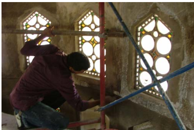
Activities and details of removing the dust and the recent limewash layer around the first level windows of the mausoleum
