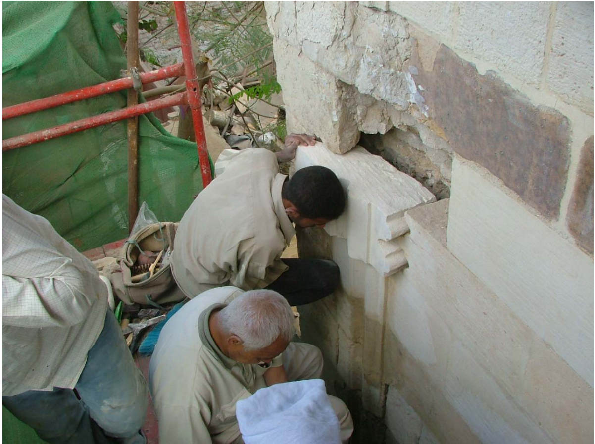
Stone replacement activities on the lower part of the west façade
