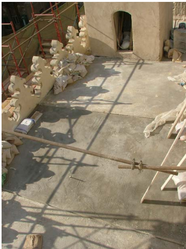
The upper insulation layer during application and after hardening
