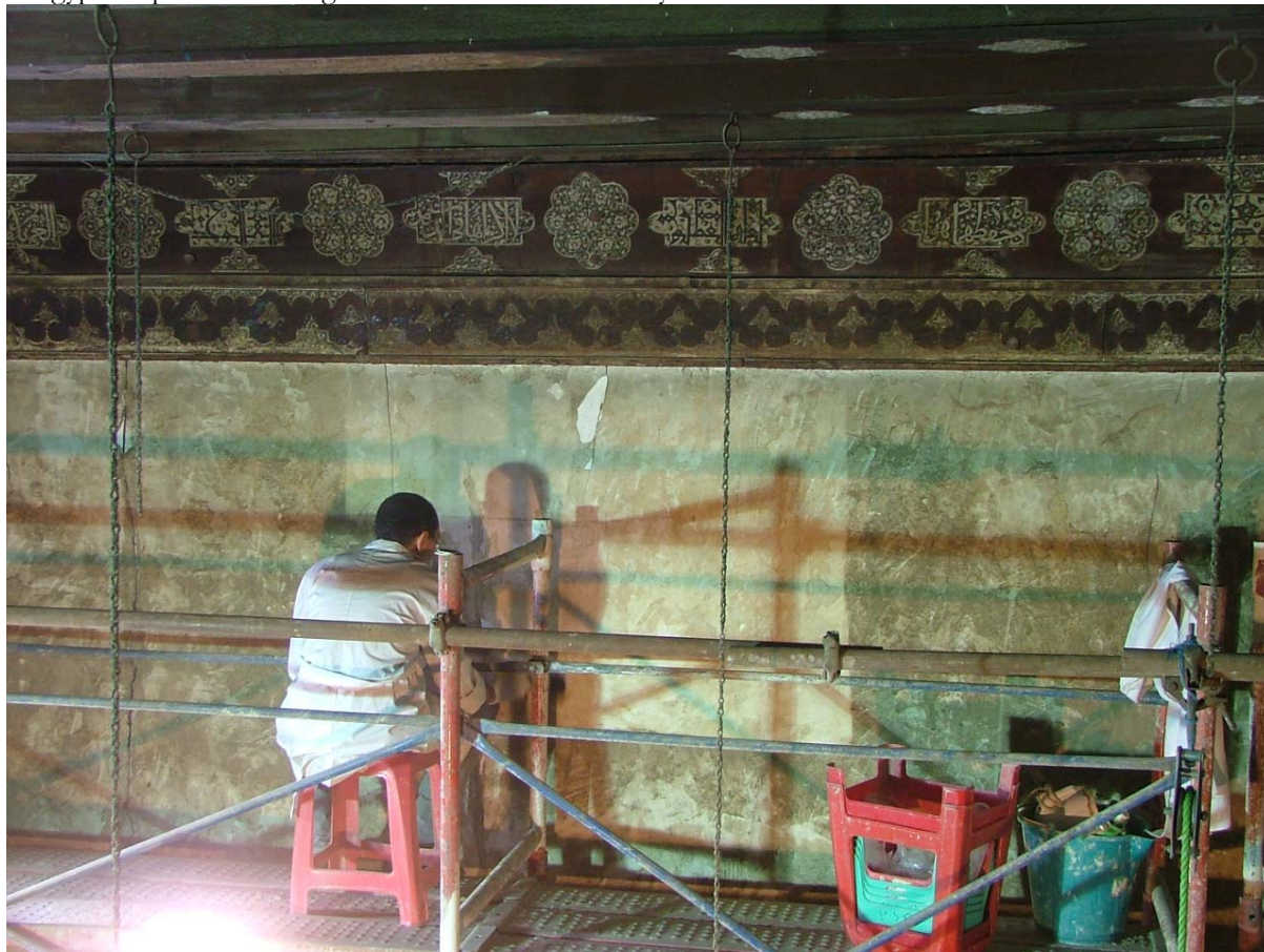
Activities of removing the fine dust from the walls (middle part cleaned; left and right still with fine dust)
