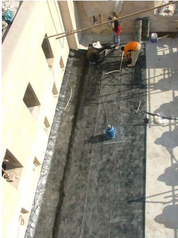
Insulation activities on the south ceiling and water testing the insulation before applying the upper mortar mix layer
