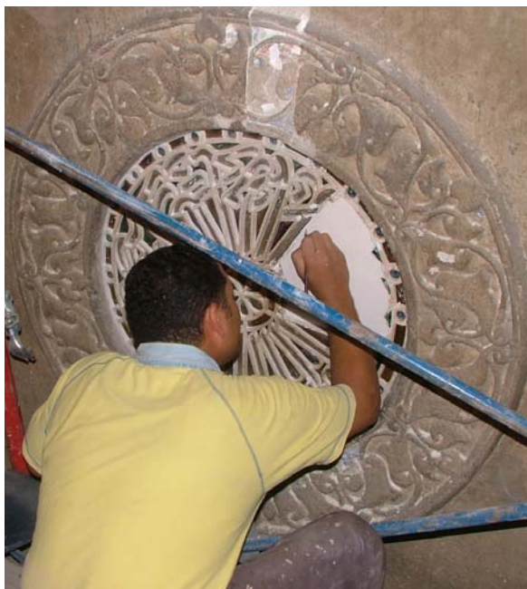
Views of repairing and protecting the gypsum decoration in-situ
