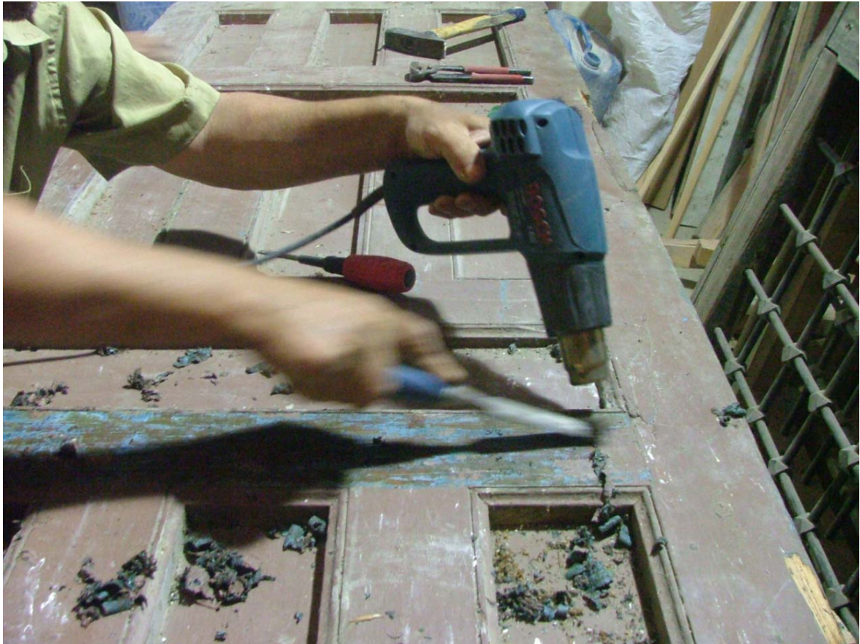
Removal of modern paint using the hot air gun
