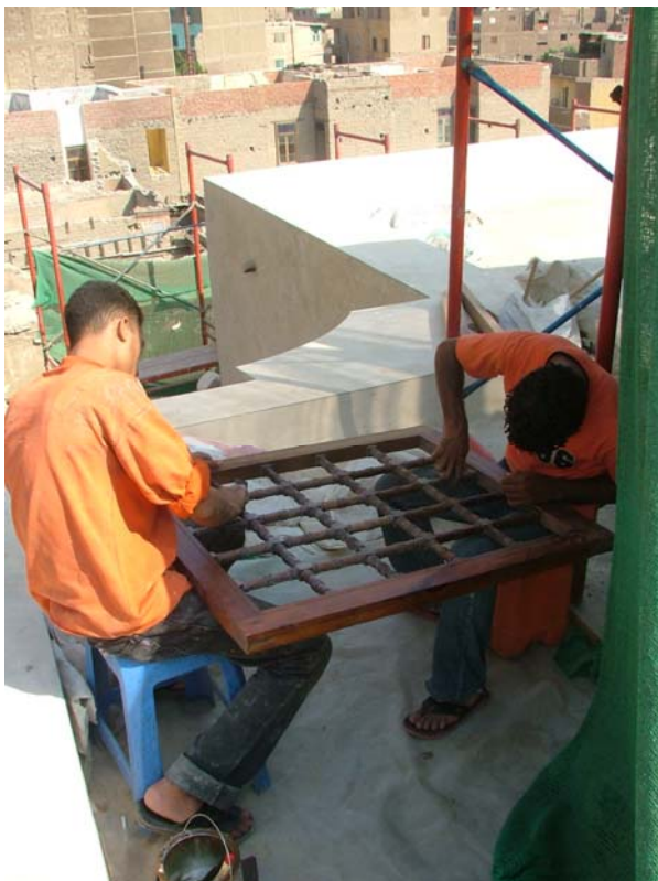
Work of painting the shokhsbaykha and its wooden screens
