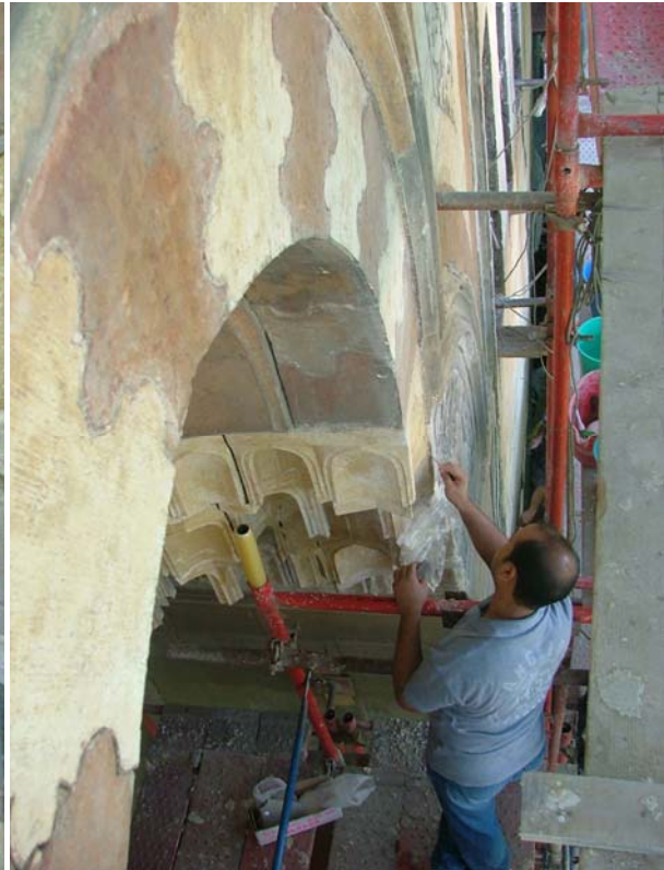
Poulticing and cleaning of the muqarnas entrance porch and its results
