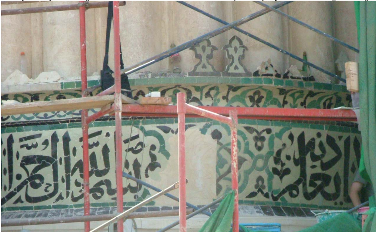
View of the crescents and the retouching tests of the floral pattern
