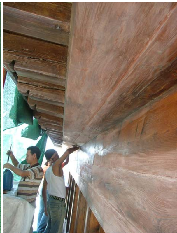
Work of painting the shokhsbaykha and its wooden screens
