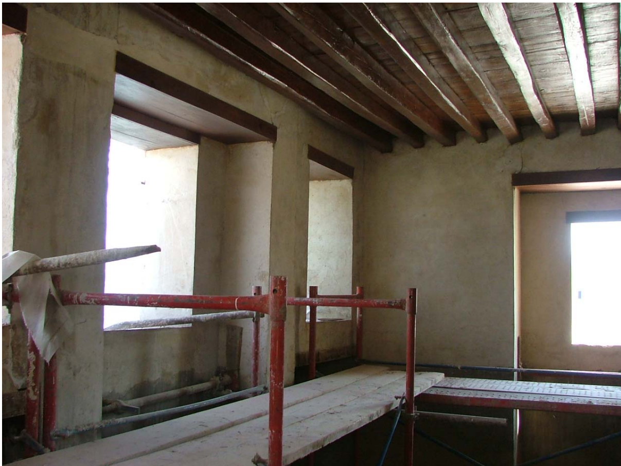
View of the upper part of room 2.2 after painting the ceiling and poulticing the walls
