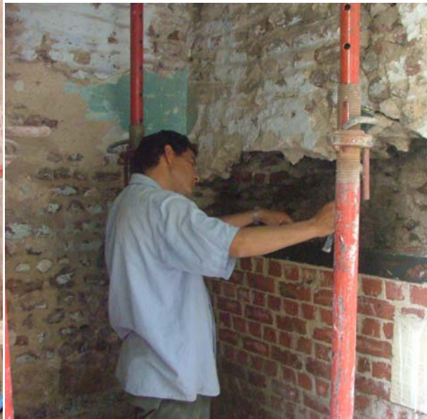
Brick repair and reconstruction activities of damaged and crumbling brick walls in the shops on the western façade
