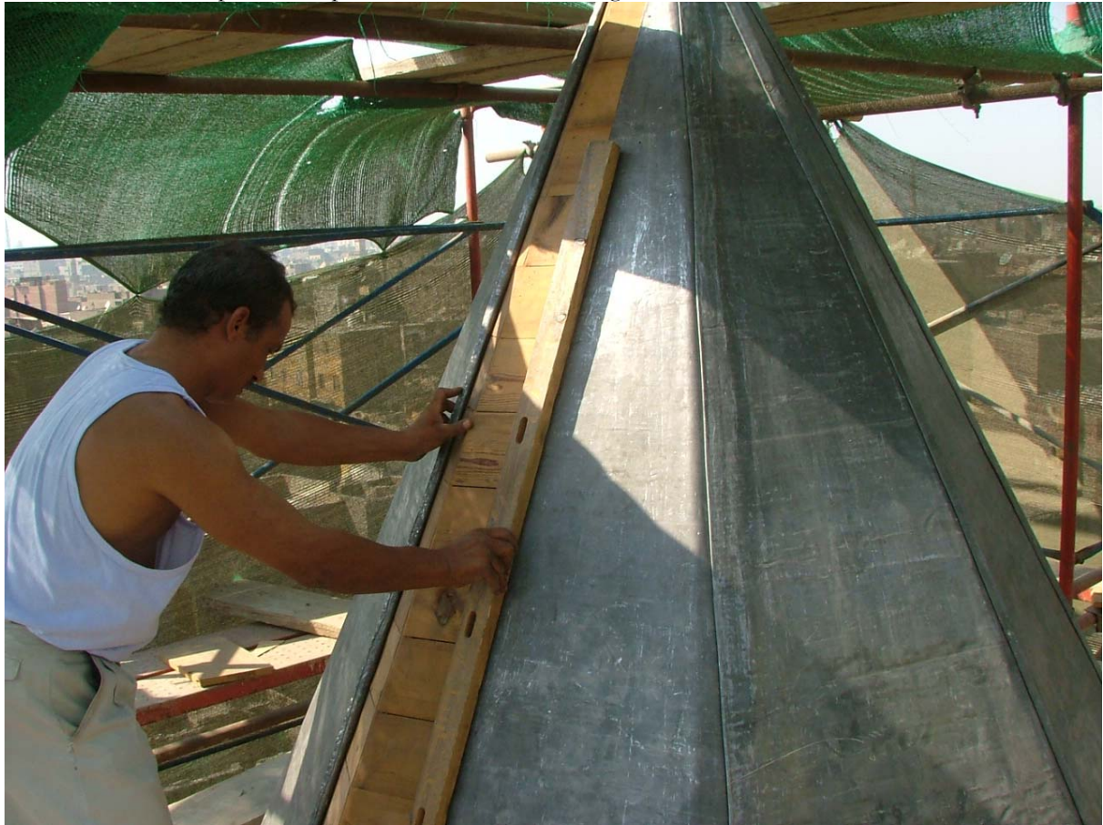
Placing the lead sheet of the insulation of the minaret
