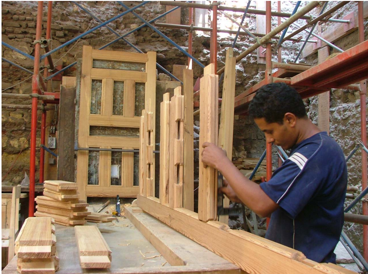
Manufacturing a new wooden door replacing the damaged one of shop 5
