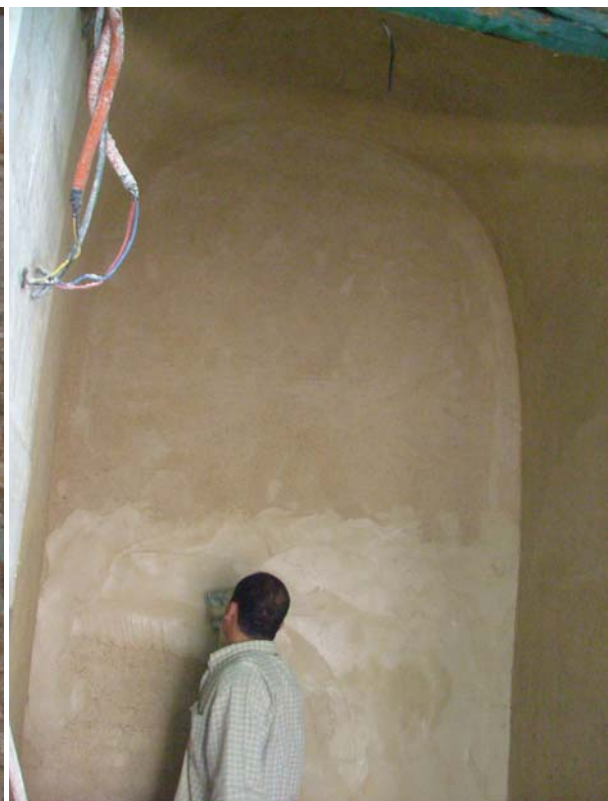
Plastering the brick walls of the shops
