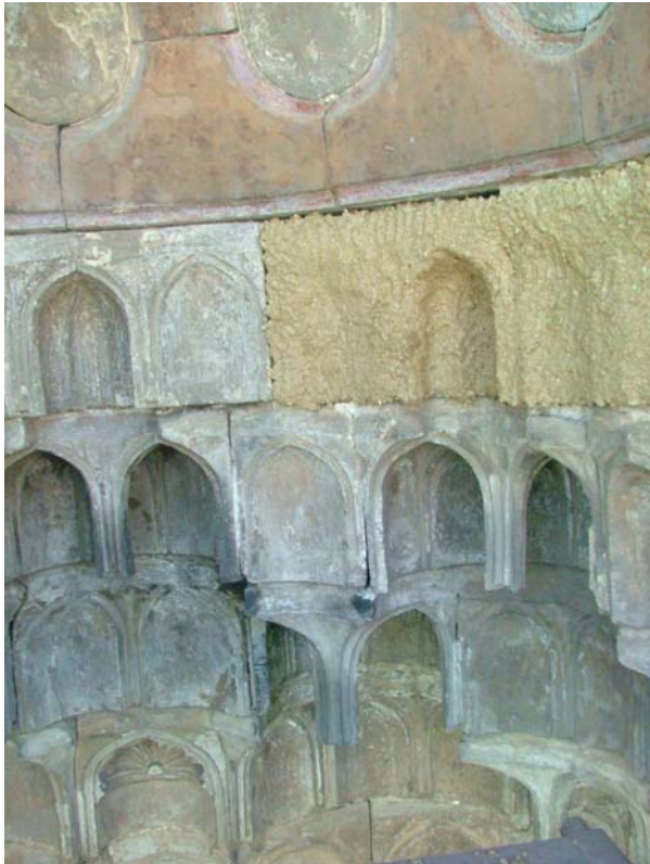
Poulticing and cleaning of the muqarnas entrance porch and its results
