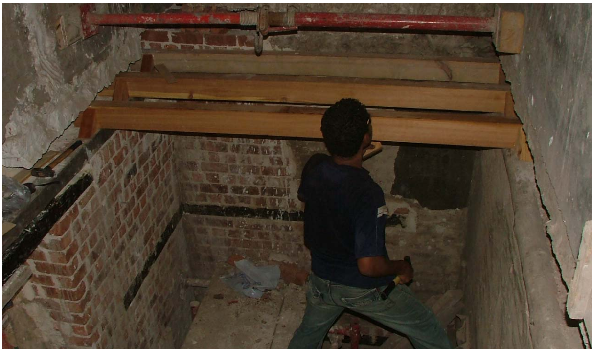
Erecting the wooden ceiling of room M1
