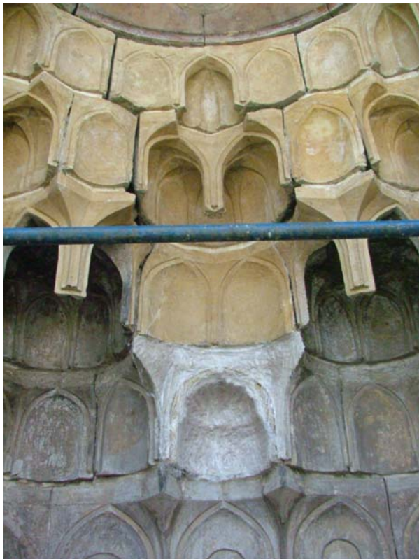
Poulticing and cleaning of the muqarnas entrance porch and its results
