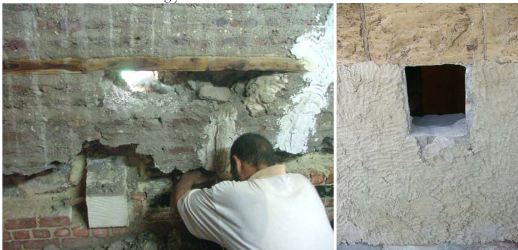
View of the interior of the room (1.2) on the western façade during brick repair activities and extending the stones into the brick wall (left photo shows the opening for the stone before placing it into the wall showing the thin thickness of the wall).
