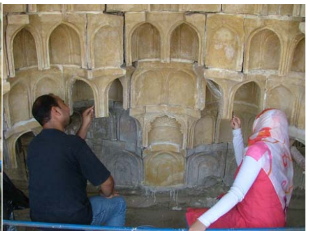
Poulticing and cleaning of the muqarnas entrance porch and its results
