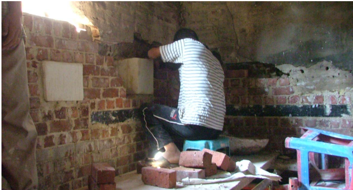
Brick repair and stitching activity in room M1
