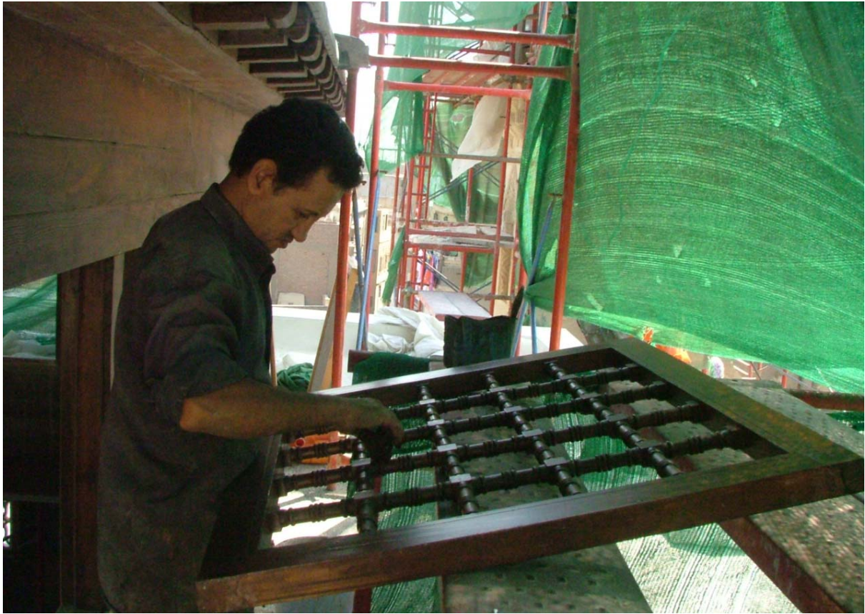
Work of painting the shokhsbaykha and its wooden screens
