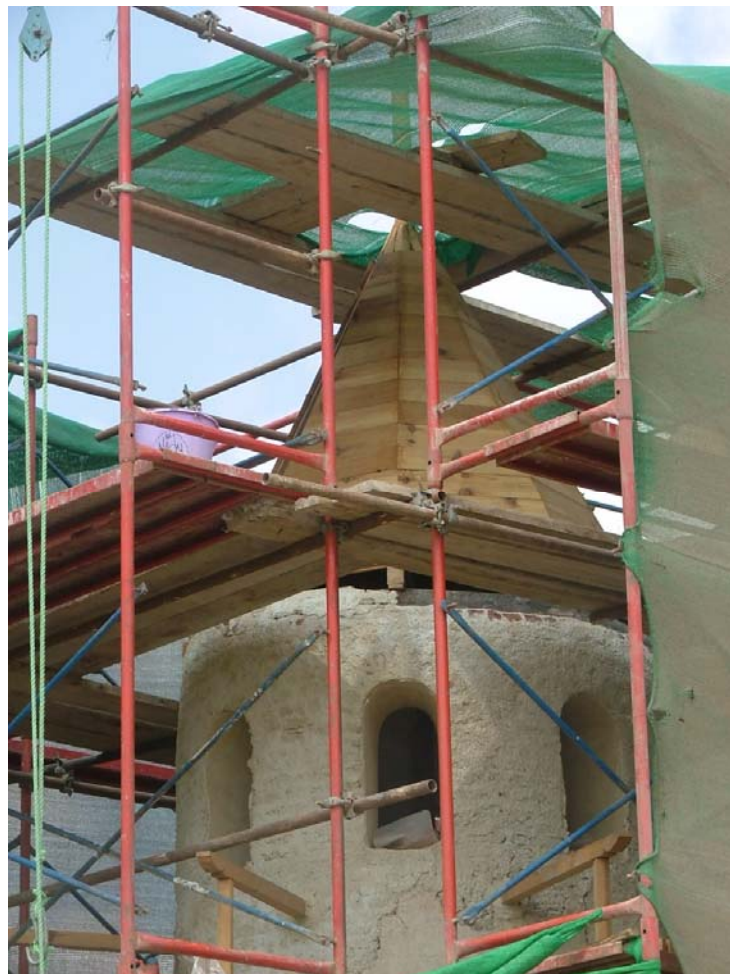
View of the minaret after the completion of the upper pencil part and during plastering activities
