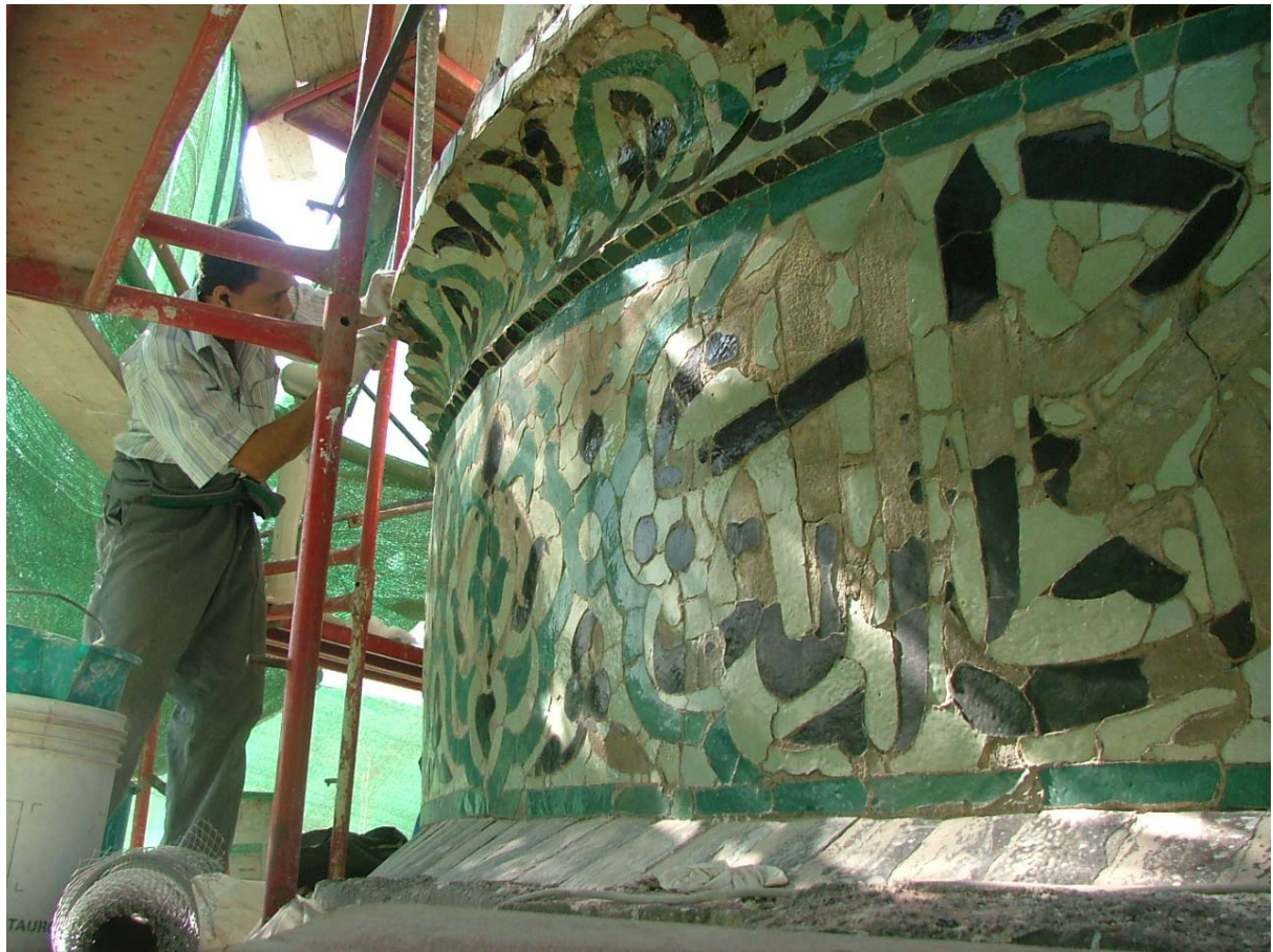
Mortar completion of the upper missing parts of the Dome Corniche
