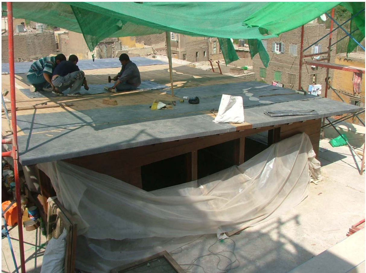
Central shokhsbekba during the insulation using lead sheets
