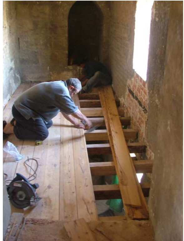
View of room 2.3 during the replacement of damaged beams and shingles.
