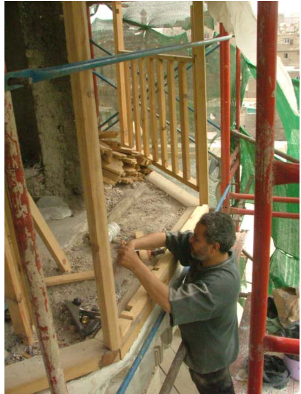
Wood manufacturing of the upper part and the surrounding handrail of the minaret balcony
