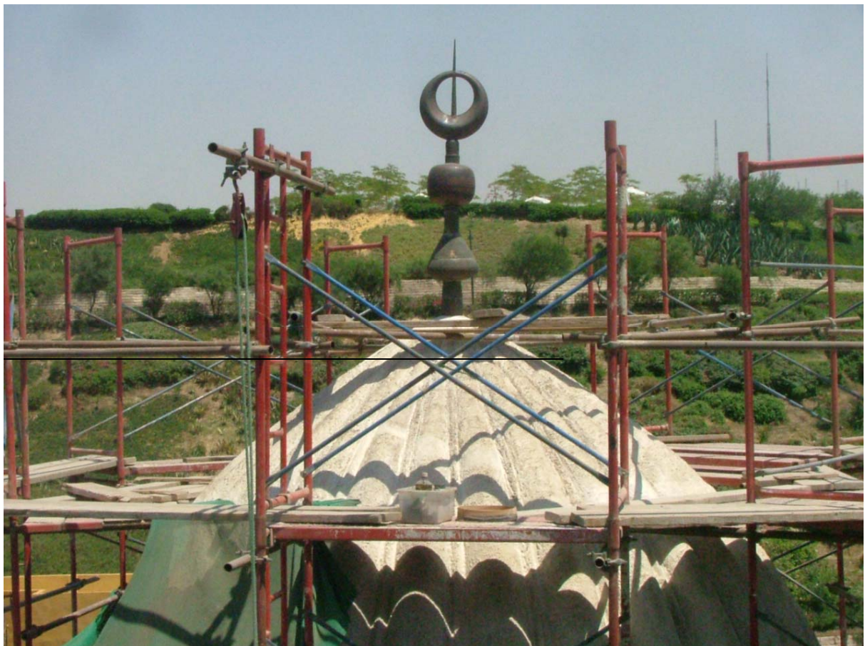
View of the dome exterior after the cleaning and installation of the copper crescent
