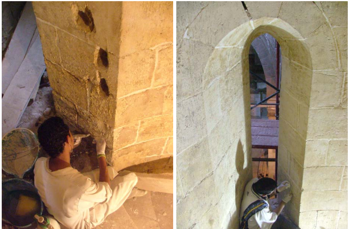
Repointing of the stone masonry after cleaning
