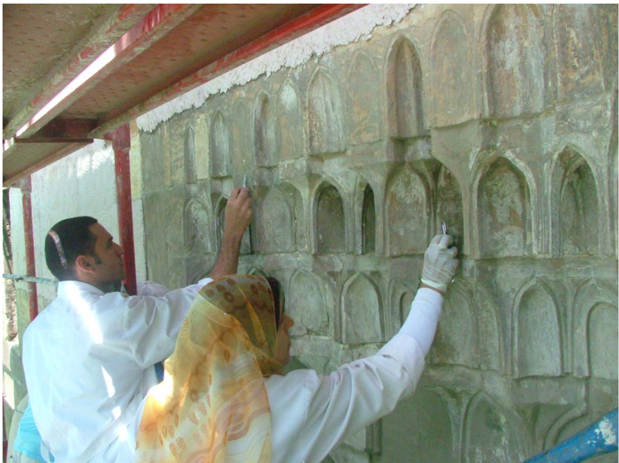
Mechanical cleaning of the western façade stalactites
