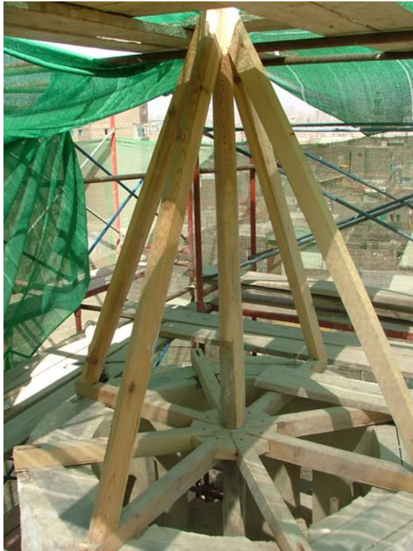
Wood manufacturing of the upper part and the surrounding handrail of the minaret balcony
