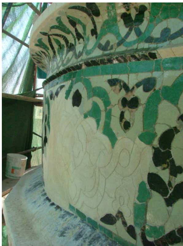
Mortar and drawing completion of missing parts
