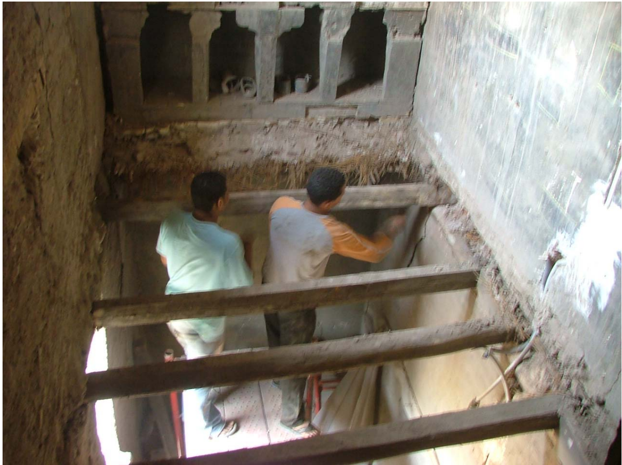
Room 1.2 during the replacement of the damaged beams
