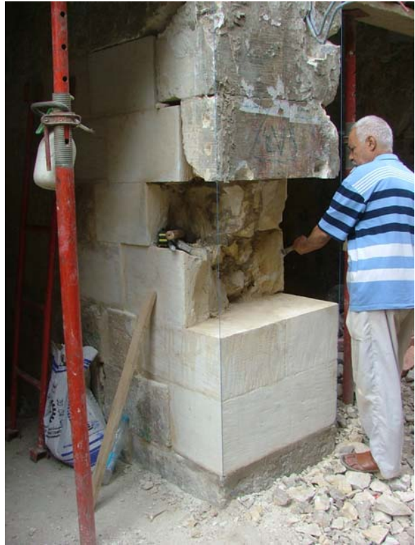
Clearing of shops on the western façade and selective replacement of damaged stones
