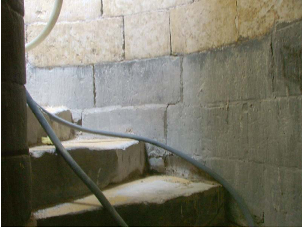
Interior of the main staircase during cleaning by sand blasting
