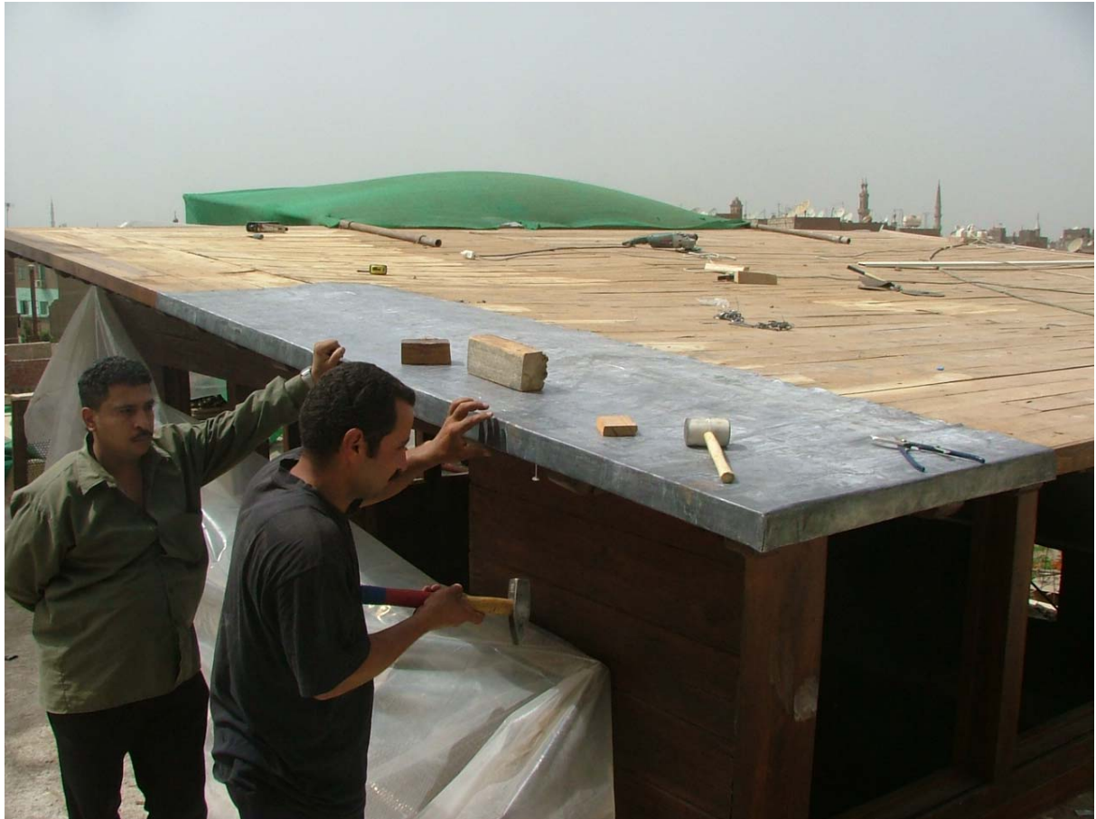
Central shokhsbekba during the insulation using lead sheets
