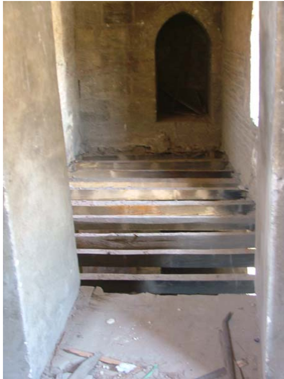
View of room 2.3 during the replacement of damaged beams and shingles.
