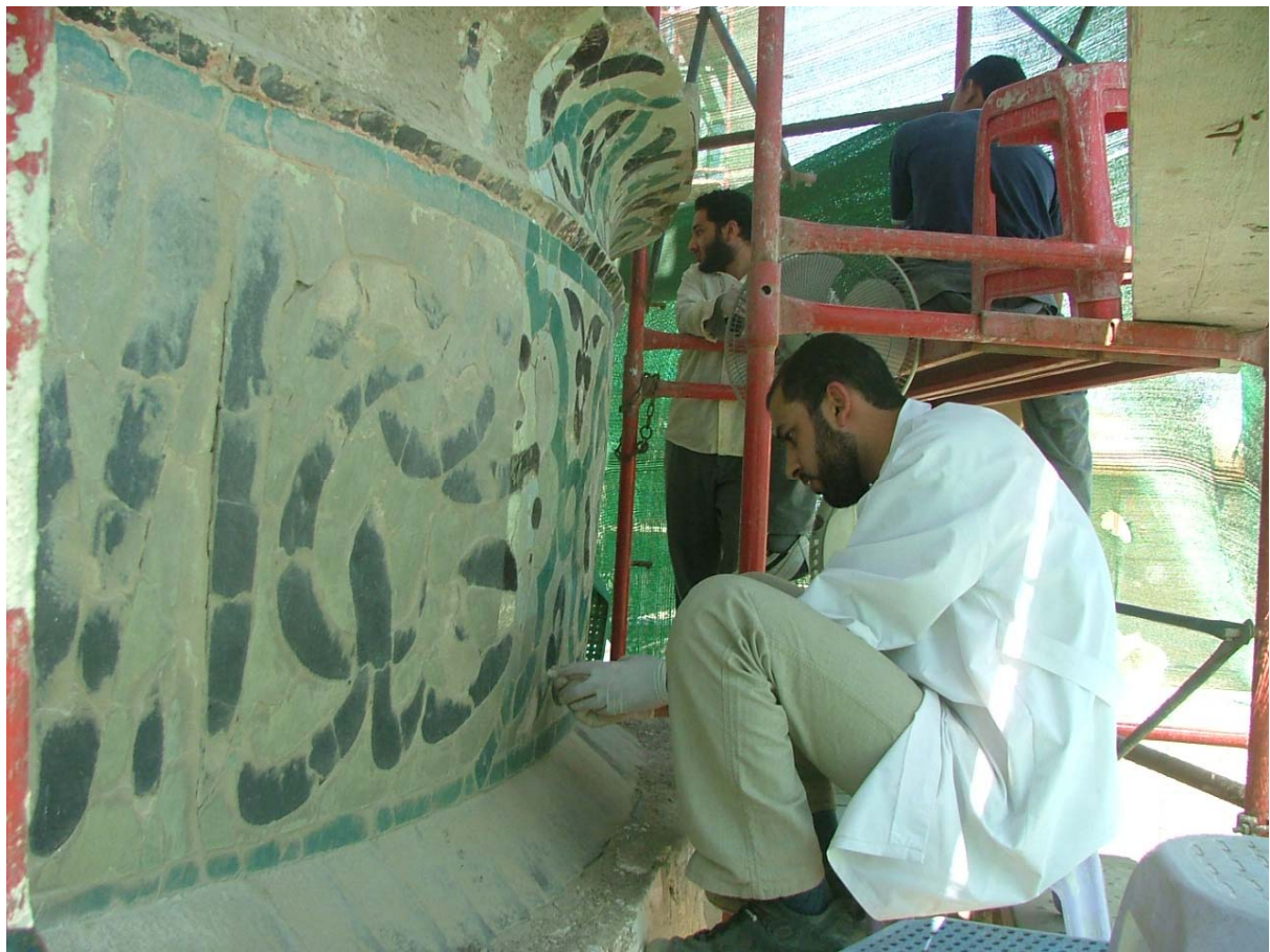
View of the ceramic inscription band on the dome during cleaning and consolidation of the ceramics
