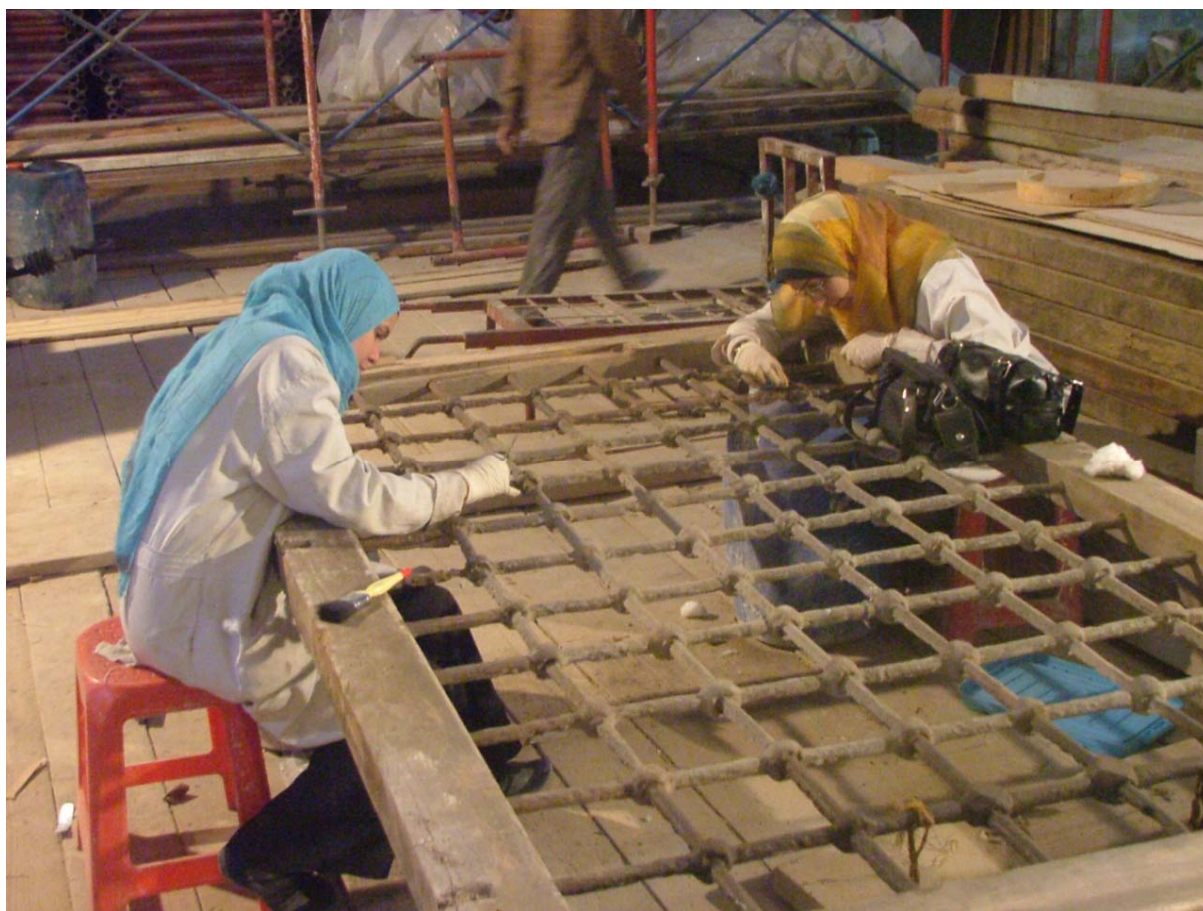
Cleaning activities of the main façade metal grill and wooden frame
