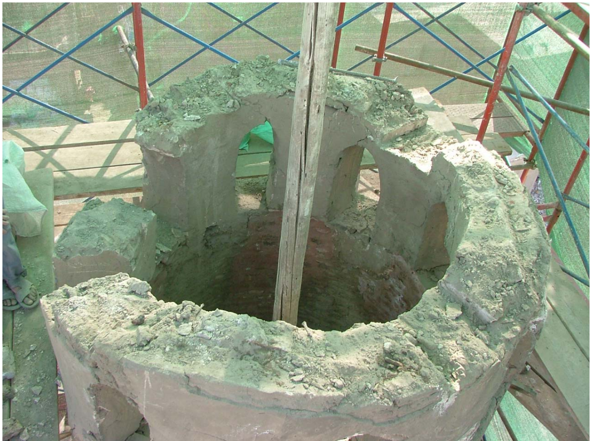
View of the minaret upper part after the removal of damaged beams.
