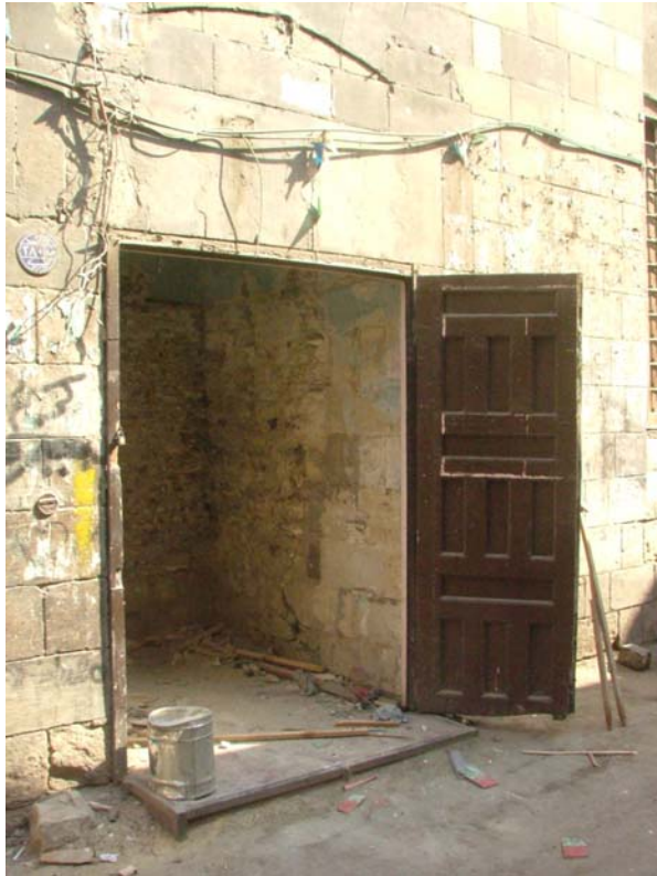
Clearing of shops on the western façade and selective replacement of damaged stones
