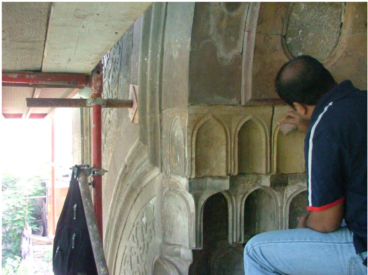
Stone cleaning activities through mechanical and poulticing techniques.
