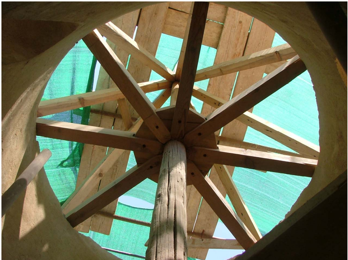
Inner view of the minaret after the installation of the main supporting beams of the upper part.
