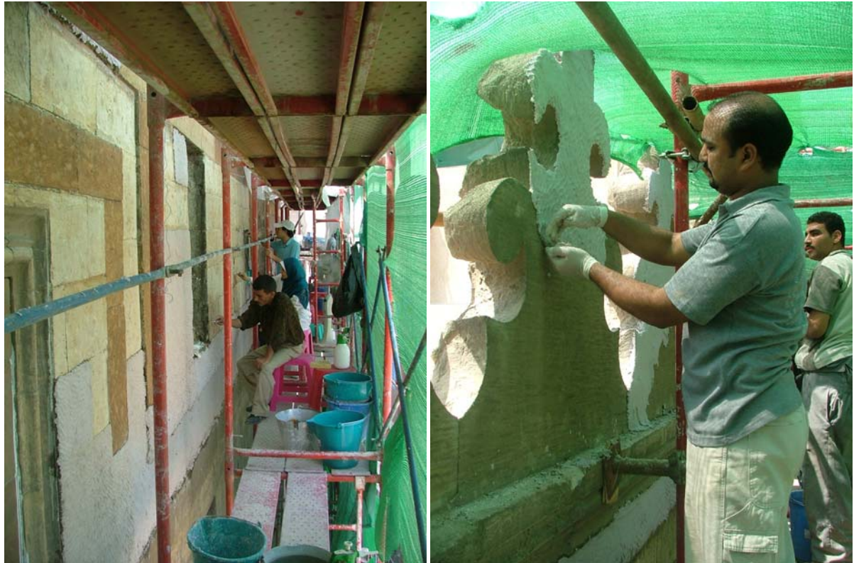
Stone cleaning activities through mechanical and poulticing techniques.
