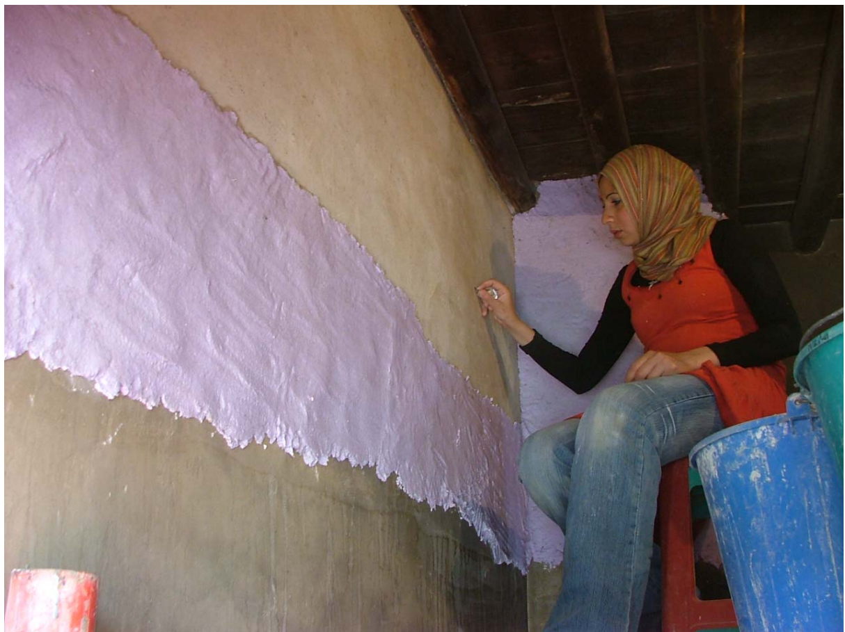
Cleaning of lime based plaster in room 2.2 using poultices after the injection of detached parts.
