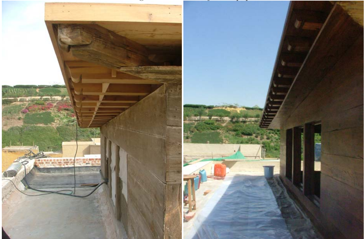
View of the central shokhsheikha after the replacement of damaged beams and shingles and after painting
