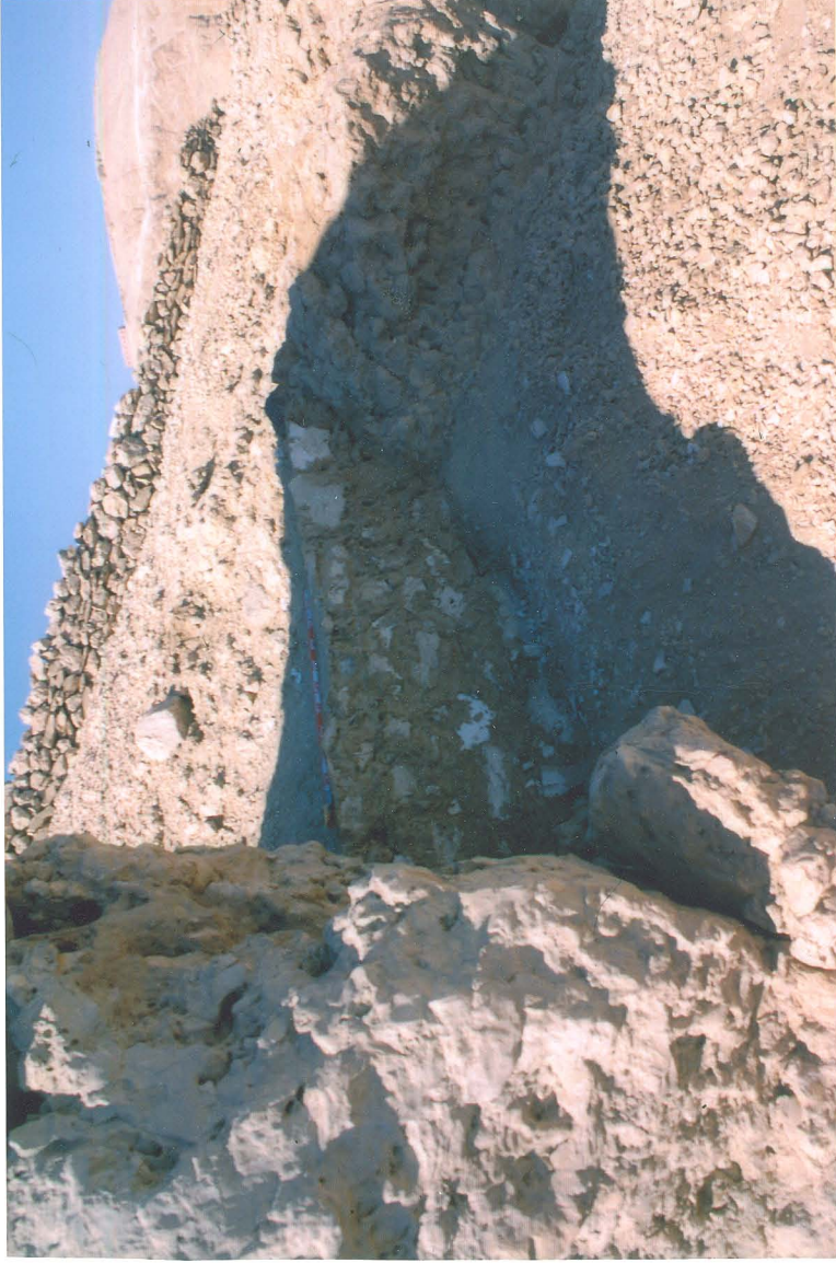
Plate 25: Two rubble walls built above the tomb to prevent the entry of rainwater, rocks and debris (photos: E.C. Brock nos. EG 20 S 235 02 and EG 12 S 253 02).
