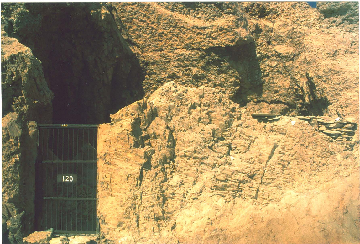
Plate 23: East wall of Inner Room, exterior, before and (above) after conservation. Photos, E.C. Brock, nos. EG 15 S 253 02, EG 1 S 252 02 .
