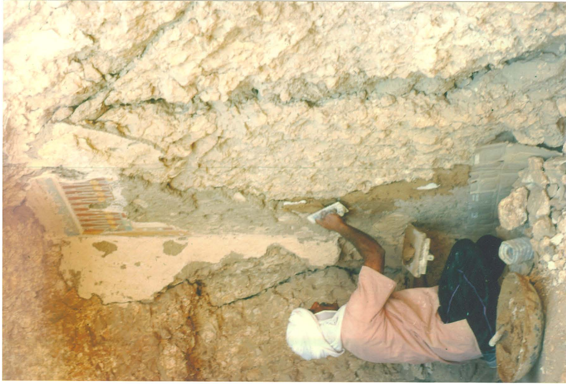
A: Mohammed 'Abd el-Warris applying mud mortar to rough rock surface of rekhyt area. (photo: L. Pinch-Brock no. EG 18 S 252 02).
